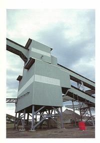
n average of 4.5 million tonnes of material is mined each year, of which 1.1 million tonnes of ore are processed. The latter is crushed and sized on an intermittent basis preparatory to the continuous process of uranium extraction.
