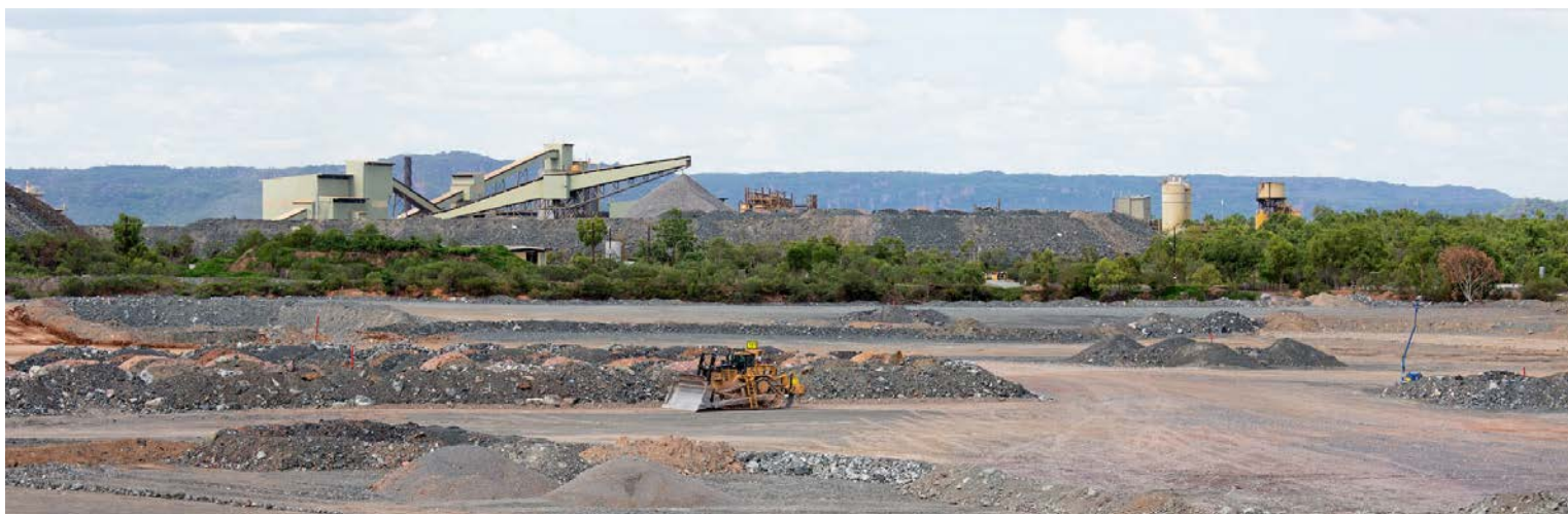
Pit 1 rehabilitation works
