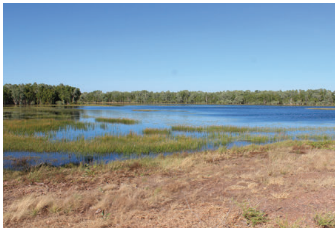
Retention Pond 1: A component of the water management system
