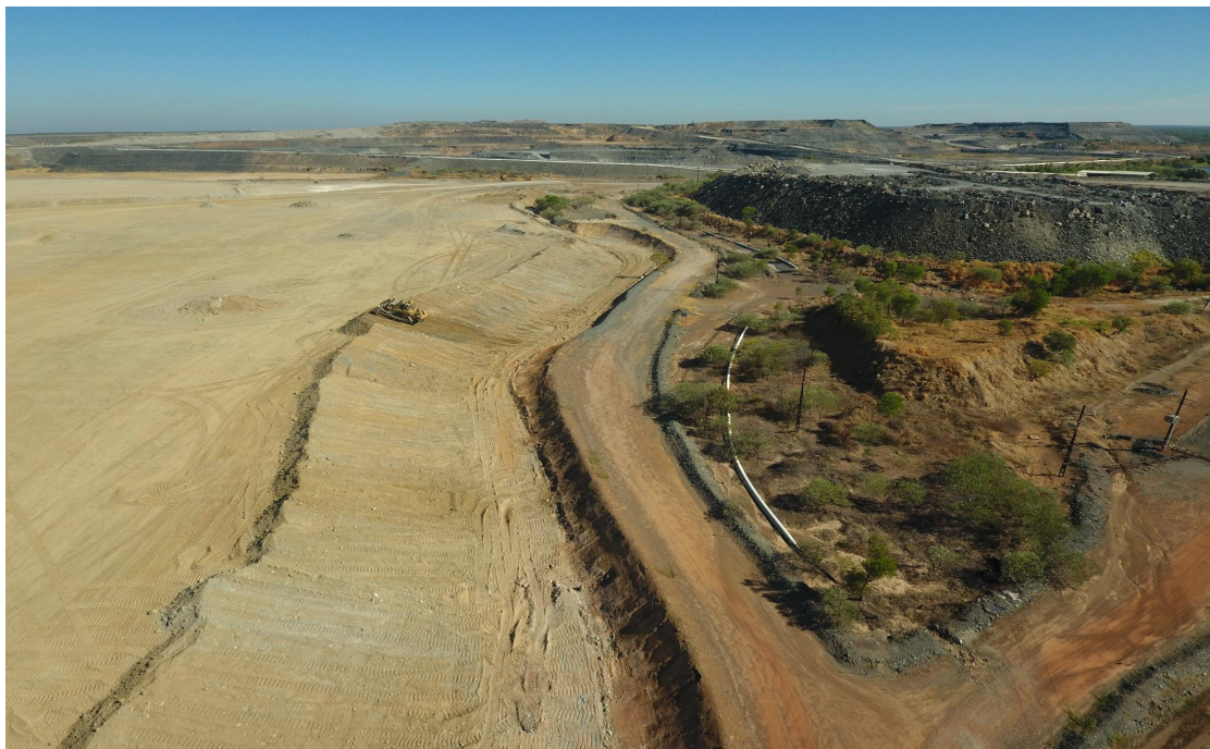
Figure 9-5: Construction of the drain at the southeast edge of Pit 1 (July 2020)
