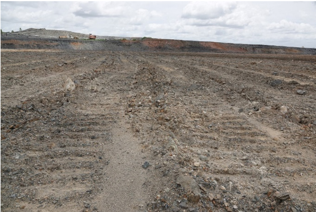
Figure 9-90: Contour ripping on Stage 13, with 3 m intervals (March 2020)
