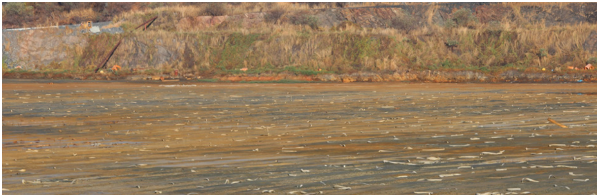
Figure 9-3: A view of some of the 7,554 vertical wick drains installed in Pit 1 in 2012
