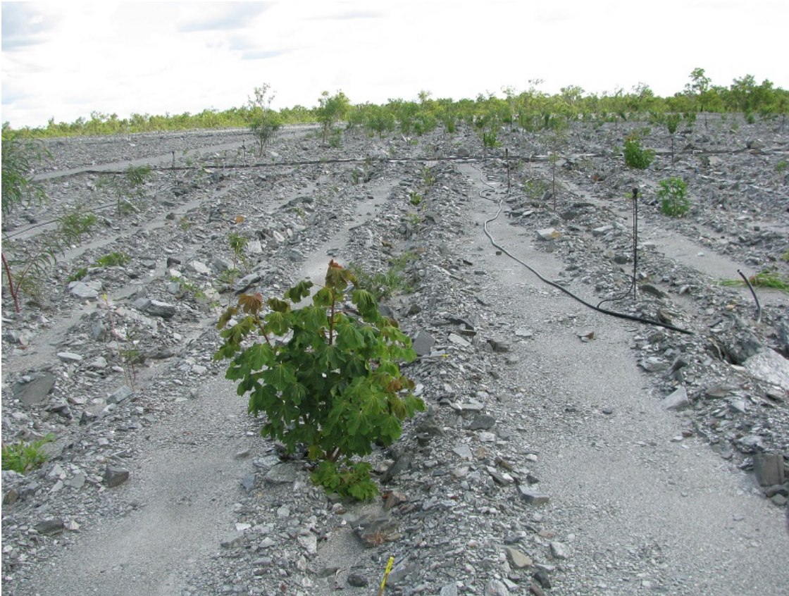
Figure 9-89: Contour ripping on trial landform trial of 2m interval (2010)
