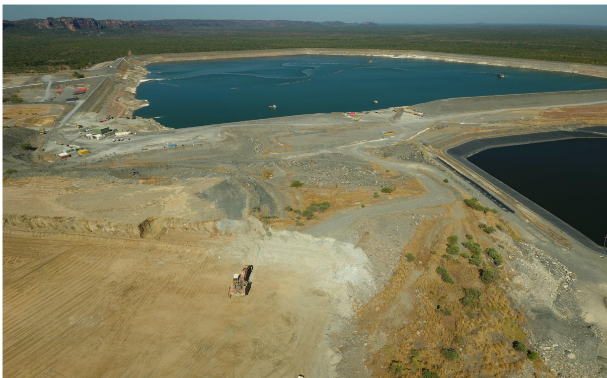
Figure 9-49: Mining Stage 10 of the stockpile area (waste is transferred to backfill Pit 1)
