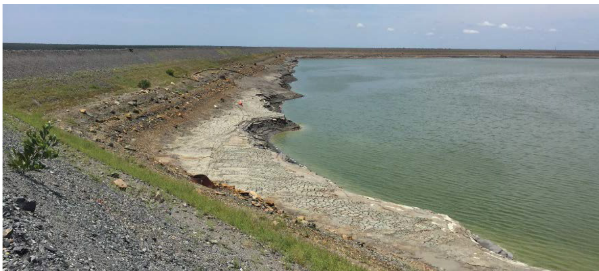
Figure 9-31: Typical remnant tailings on TSF wall after dredging
