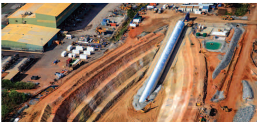
Figure 9-61: Boxcut and portal, completed in December 2012
