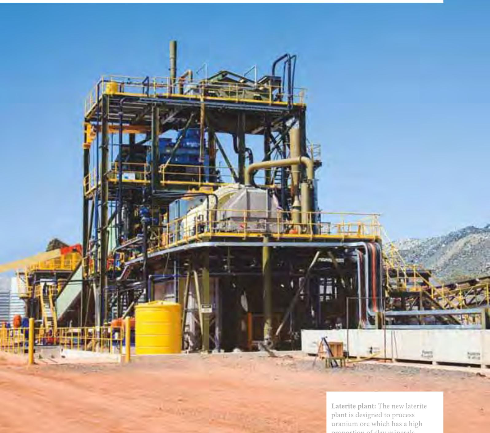
**Laterite plant:** The new laterite plant is designed to process uranium ore which has a high proportion of clay minerals.
