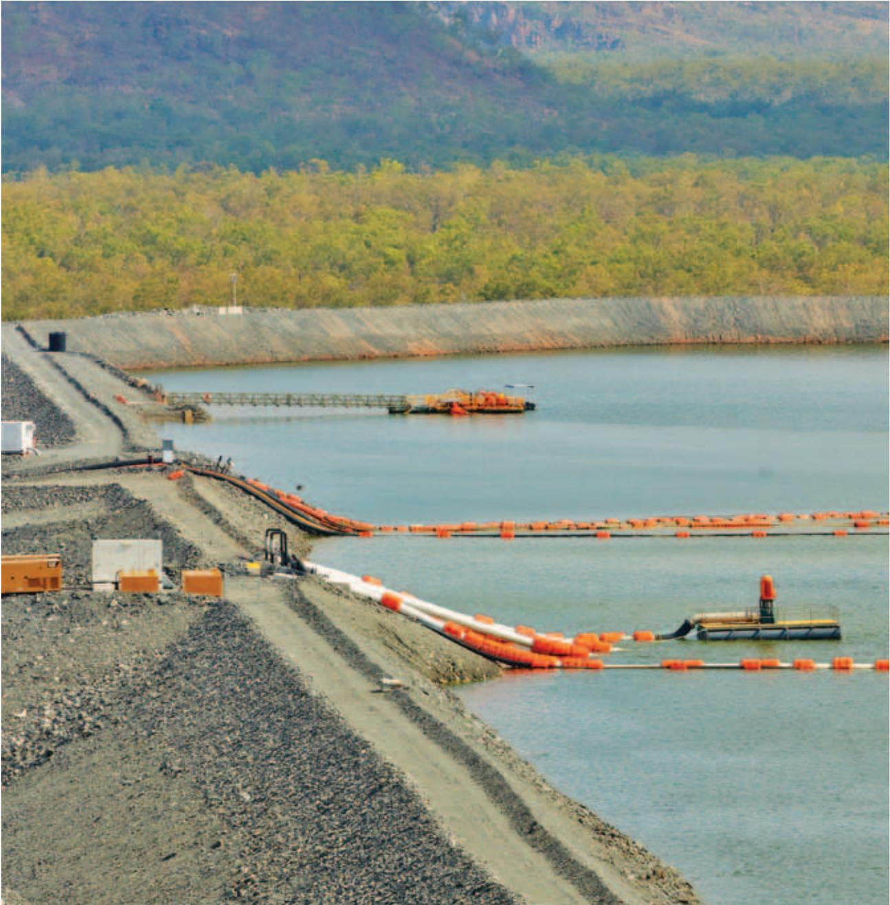
*The Tailings Storage Facility at Ranger mine stores tailings and water that has come into contact with the mine's uranium extraction circuit.*
