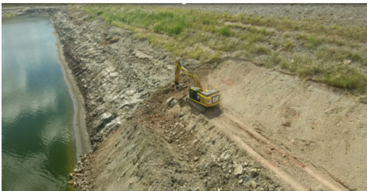
Figure 9-32: Land based excavator cleaning tailings off North wall of TSF
