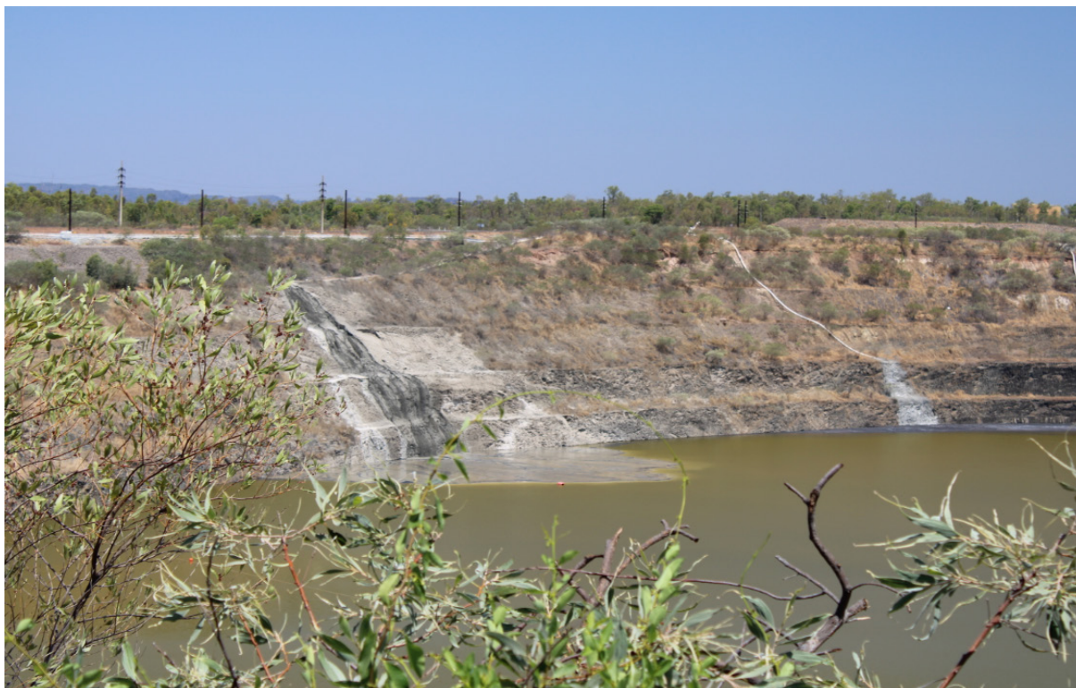
Figure 9-19: Southeast wall of Pit 3 – subaerial discharge point for mill tailings (Nov 2019)
