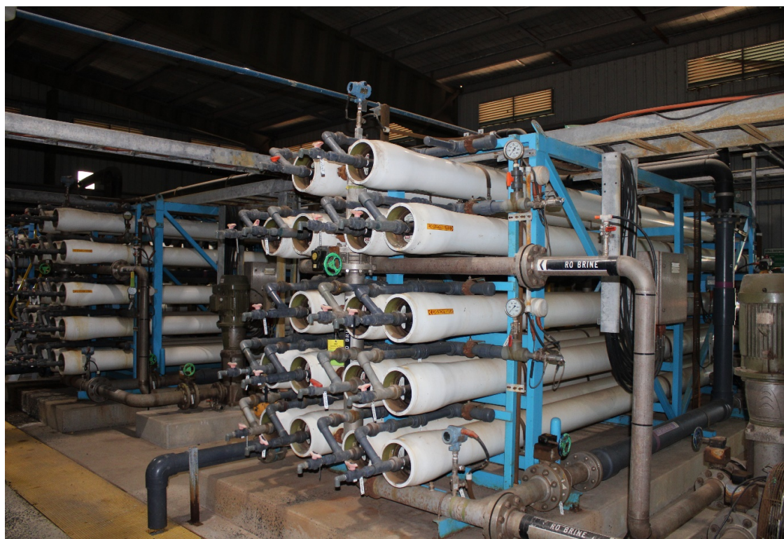
Figure 9-79: WTP 1 – reverse osmosis membranes
