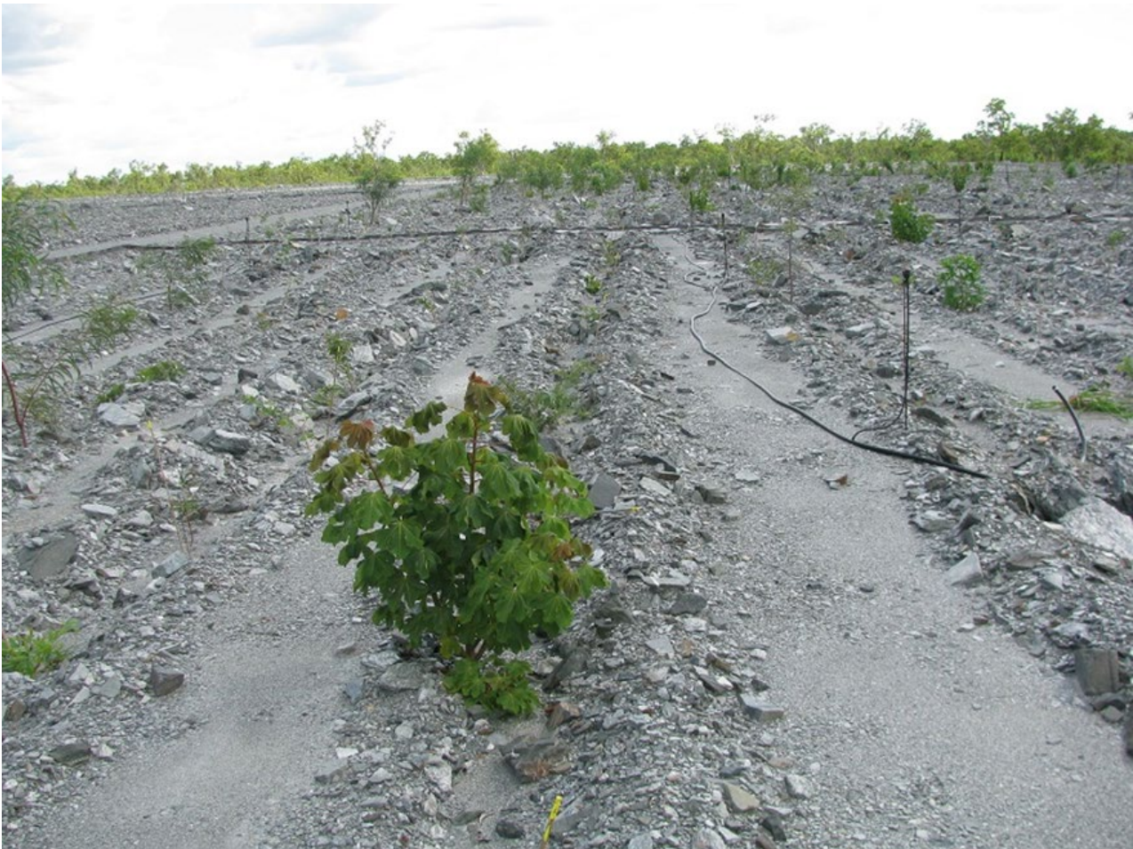
Plate 1: Contour ripping on trial landform trial of 2 m interval (2010)
