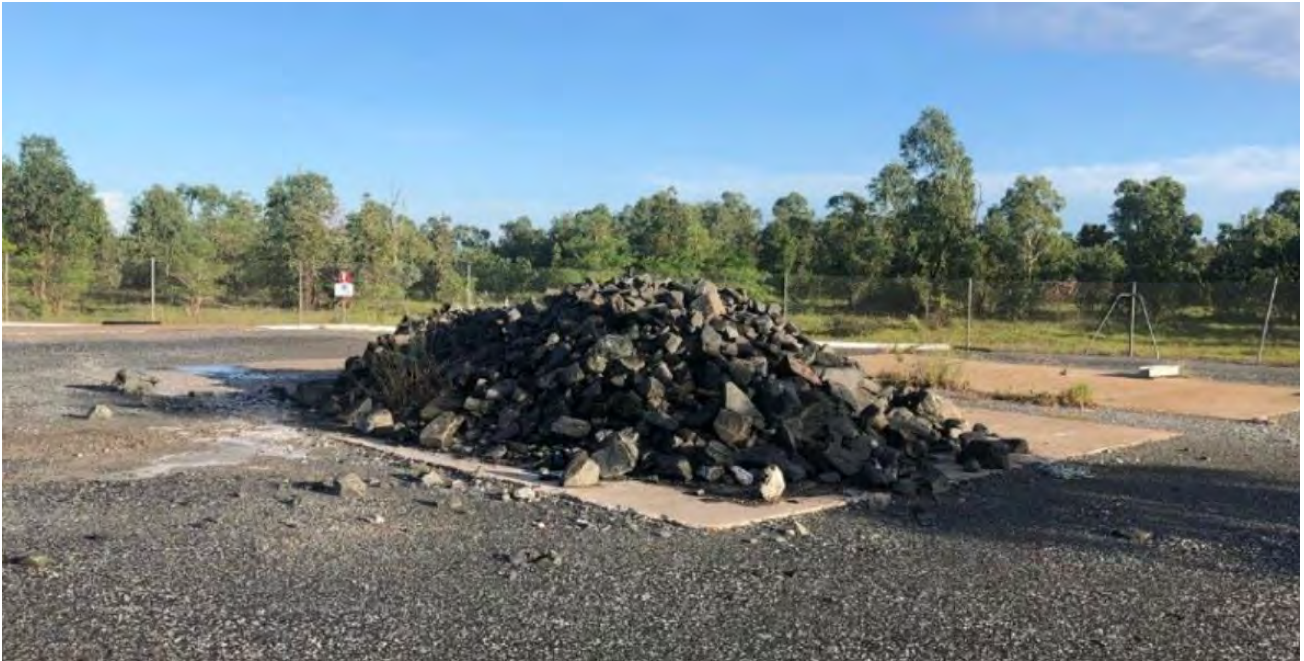
Photo 4-29: Coarse rockfill placed on top of the backfilled R3 Deeps ventilation shaft
