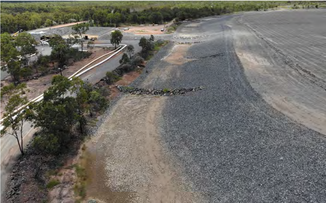
Photo 4-5: View of the perimeter drain and rock check dams along the south-east edge of Pit 1 (January 2021)
