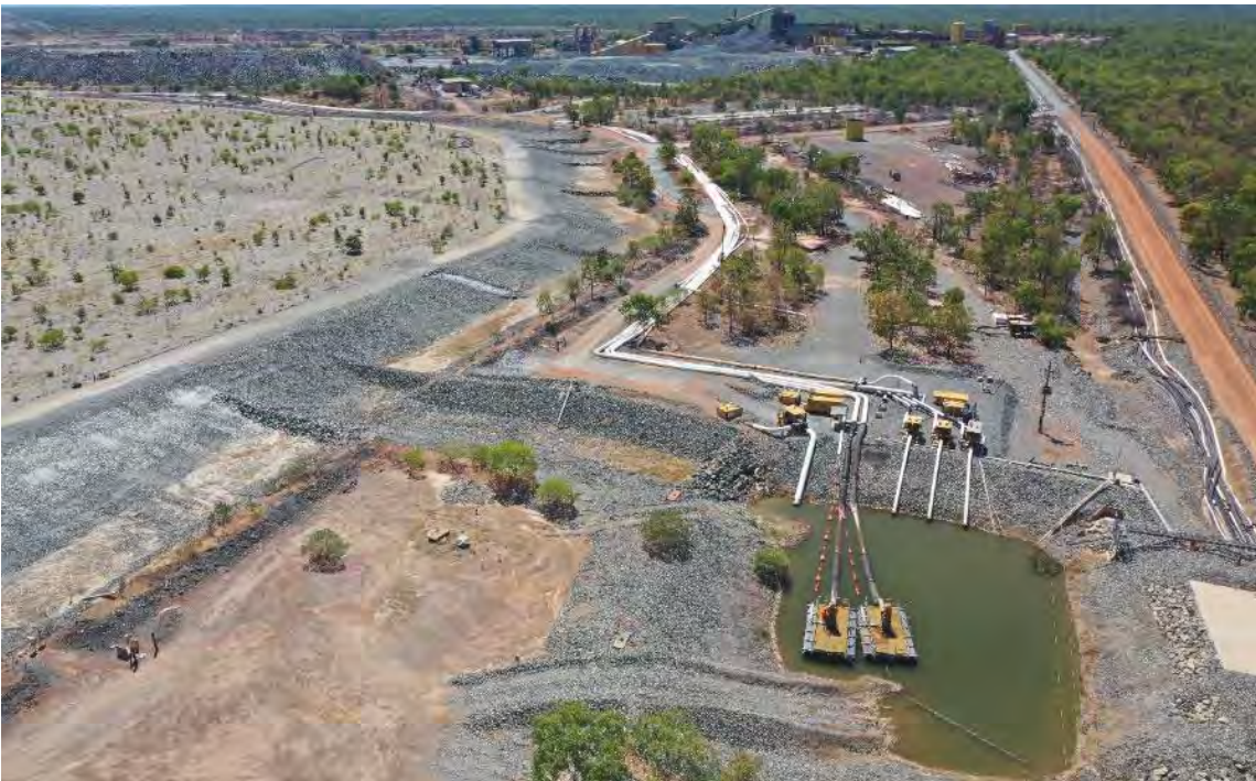
Photo 4-6: Completed Corridor Road Sump upgrade works with pumping infrastructure installed
