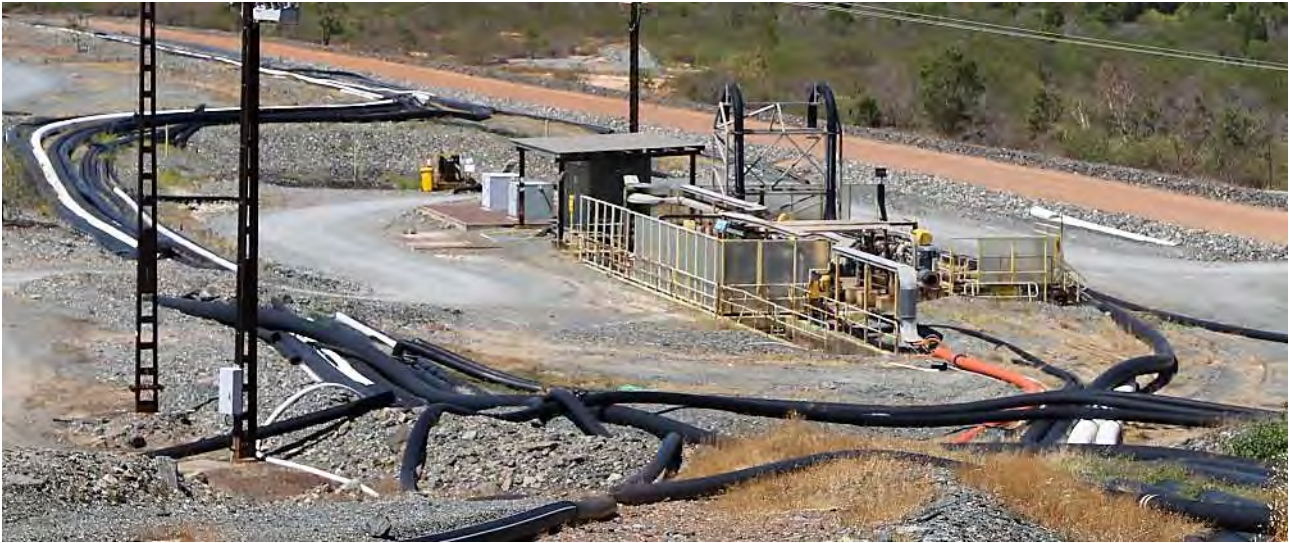
Photo 4-11: Decommissioned pumping booster station
