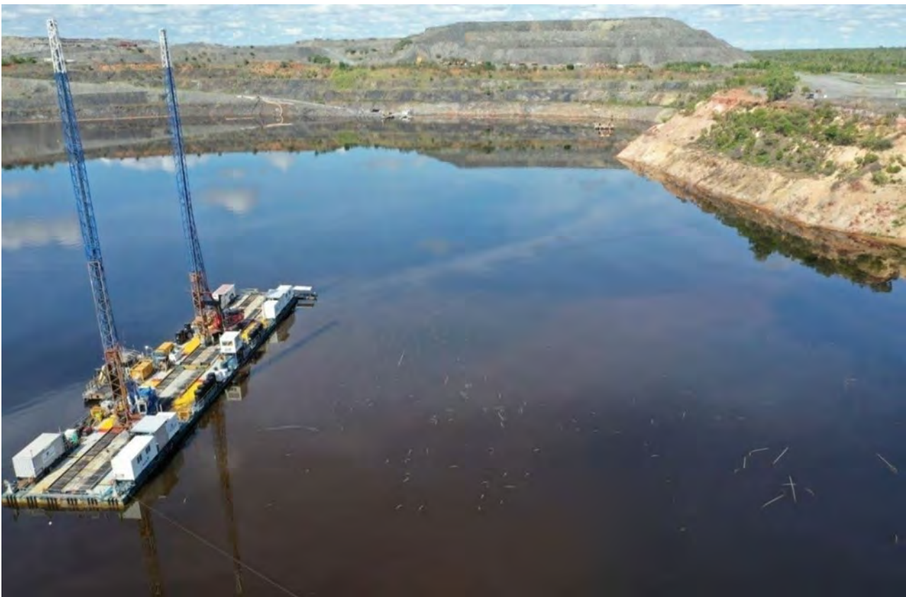
Photo 4-14: Pit 3 wicking barge and rigs
