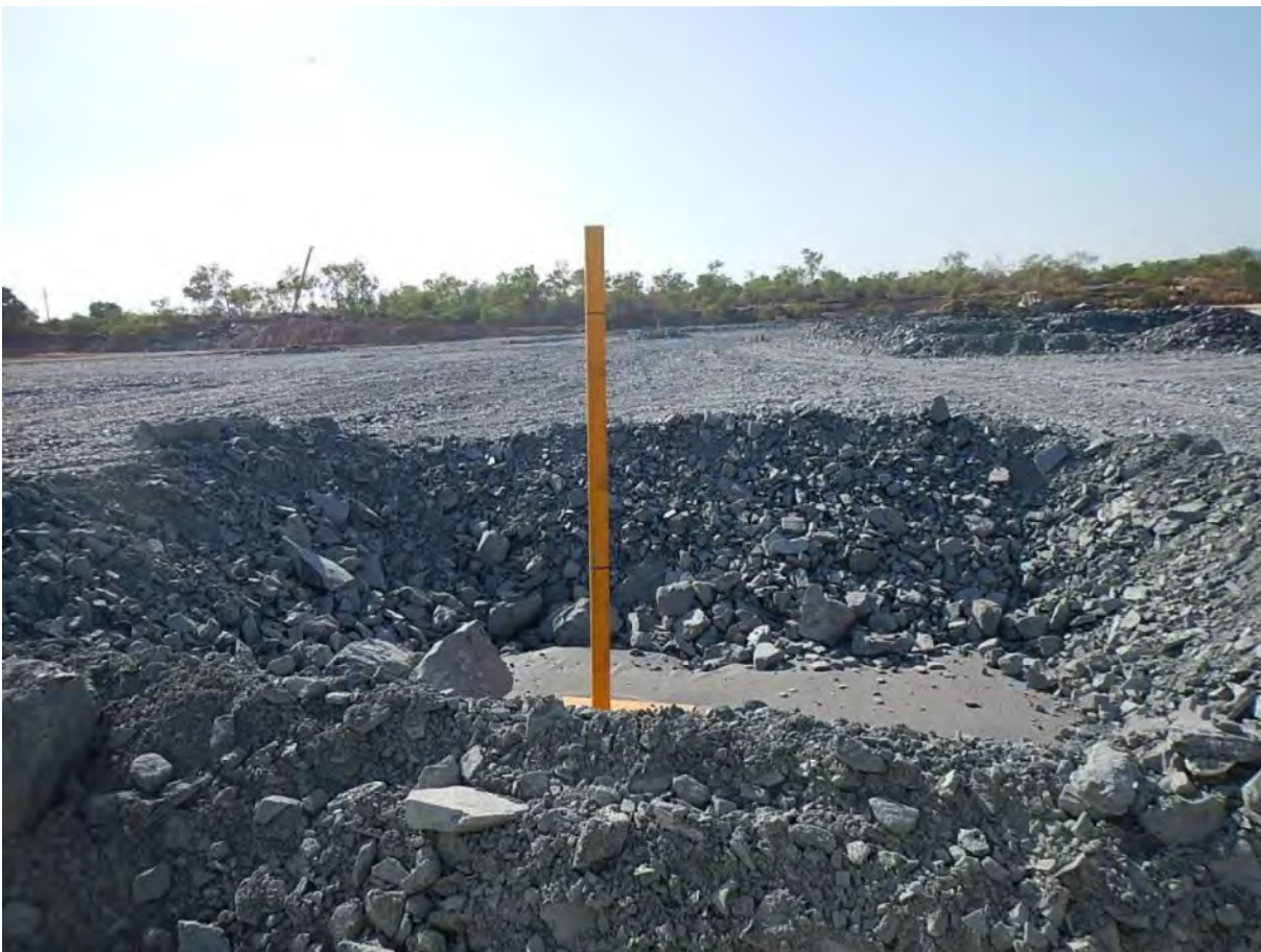
Photo 4-2: Settlement monitoring plate, with standpipe, at time of installation
