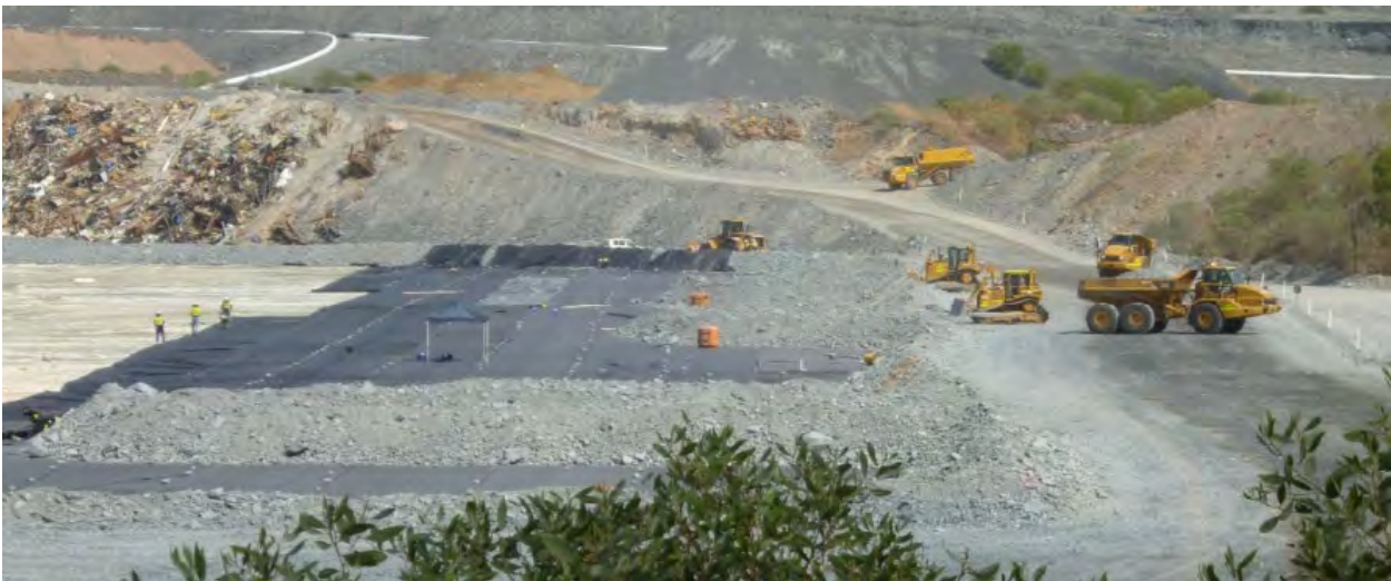
Photo 4-18: Installation of geotextile, construction of groynes and initial capping on Pit 1
