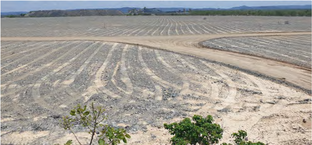
Photo 4-4: Scarification of the surface on Pit 1 (October 2020)
