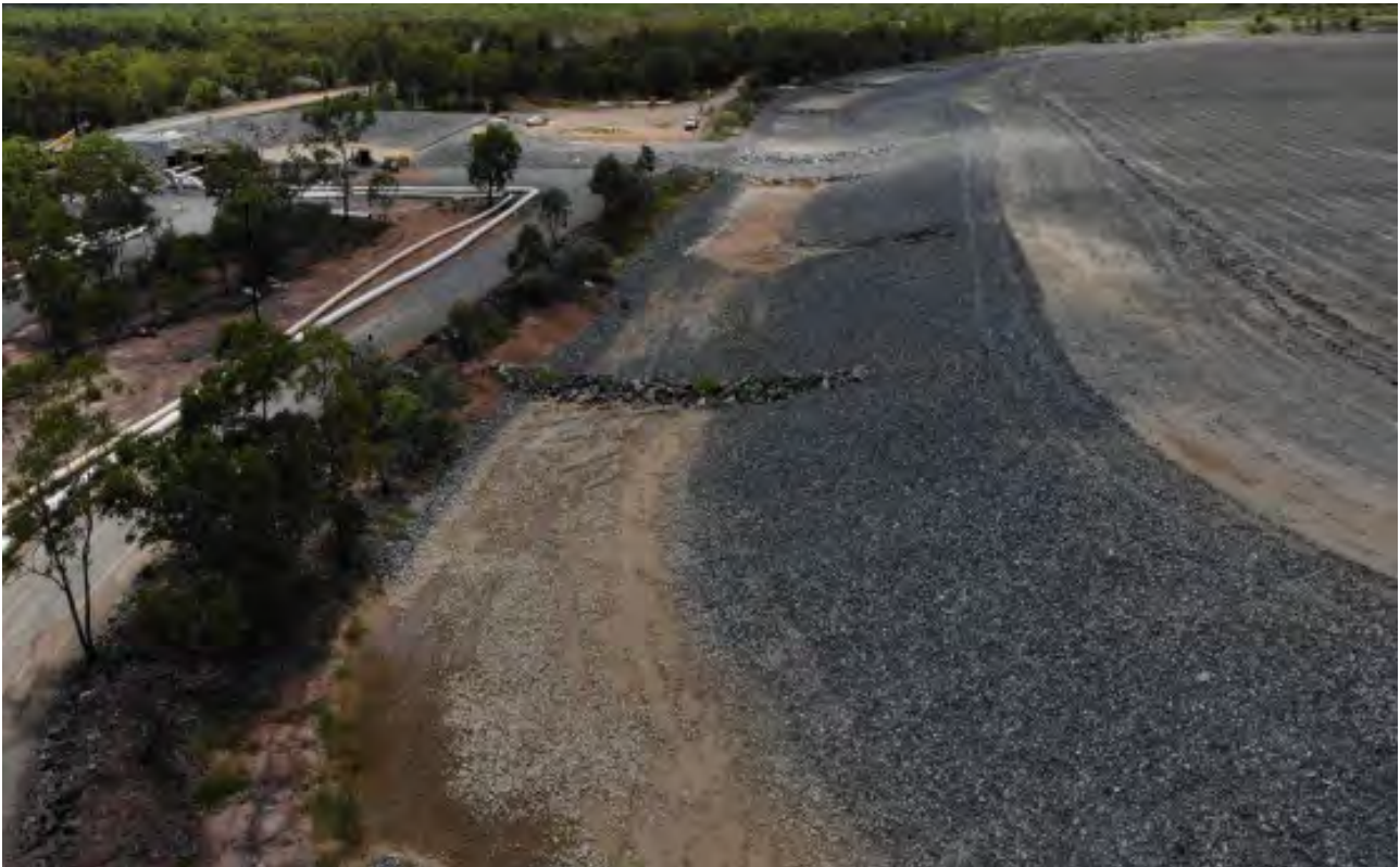
Photo 6-1: Pit 1 perimeter drain with sediments visible behind rock check dams
