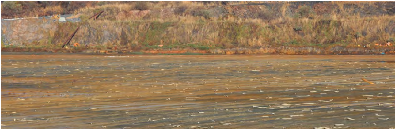
Photo 4-3: Tailings surface showing tops of vertical wick drains installed in Pit 1
