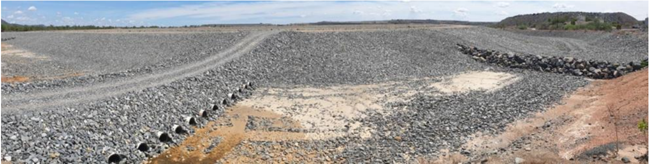
Photo 8: Pit 1 perimeter drain with access track (left) and rock check dam (right) (2021)
