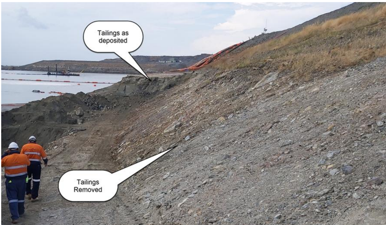
Photo 15: Cleaning remnant tailings from walls of tailings storage facility (2020)
