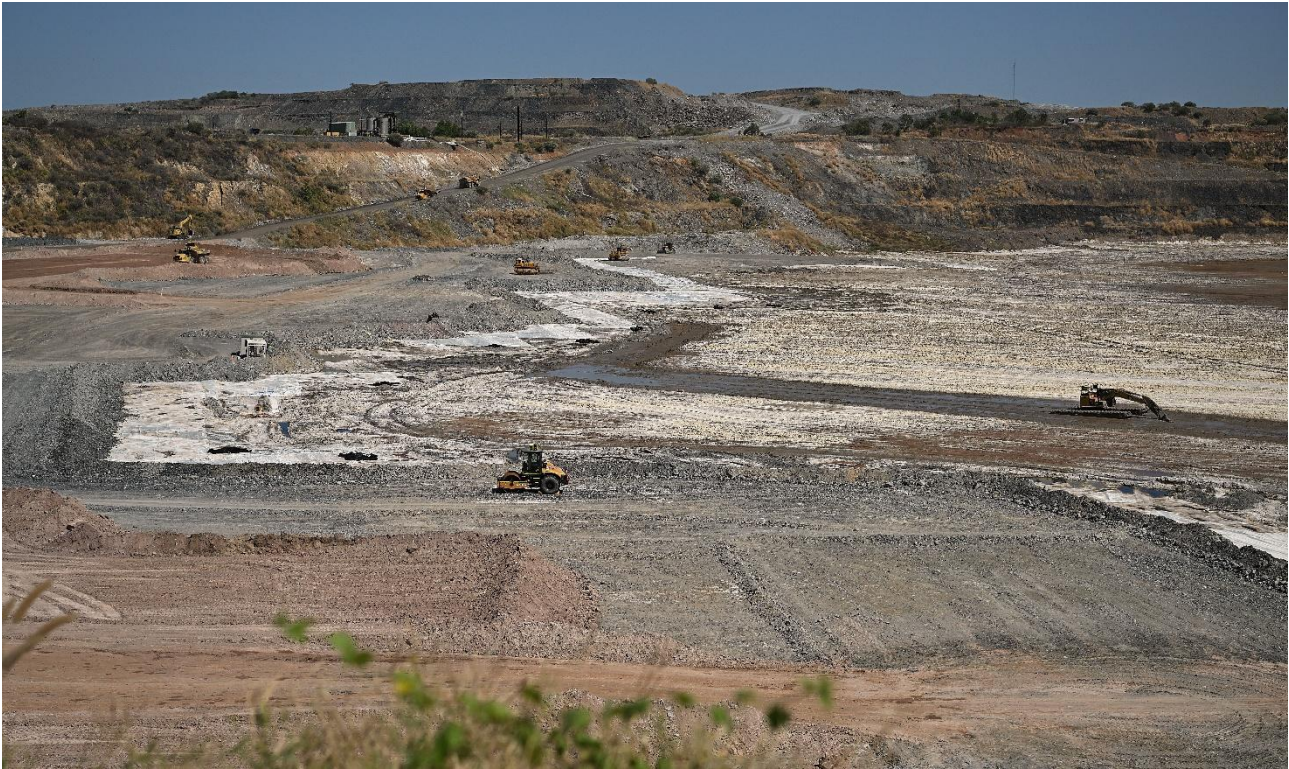
Photo 14: Installation of geotextile and construction of initial capping on Pit 3 (2025)
