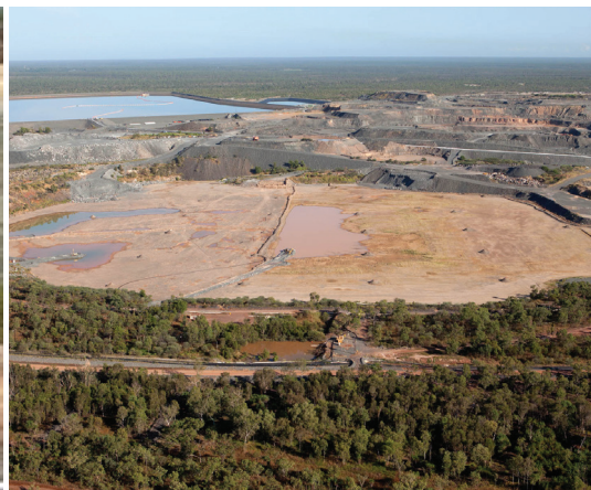
Pit 1 2016 – initial tailings cover complete
