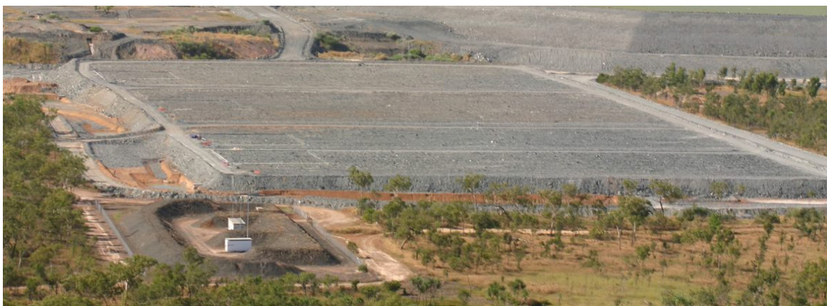
Plate ES15: Ranger Water Dam in final stages of remnant tailings removal from floor (2021)
