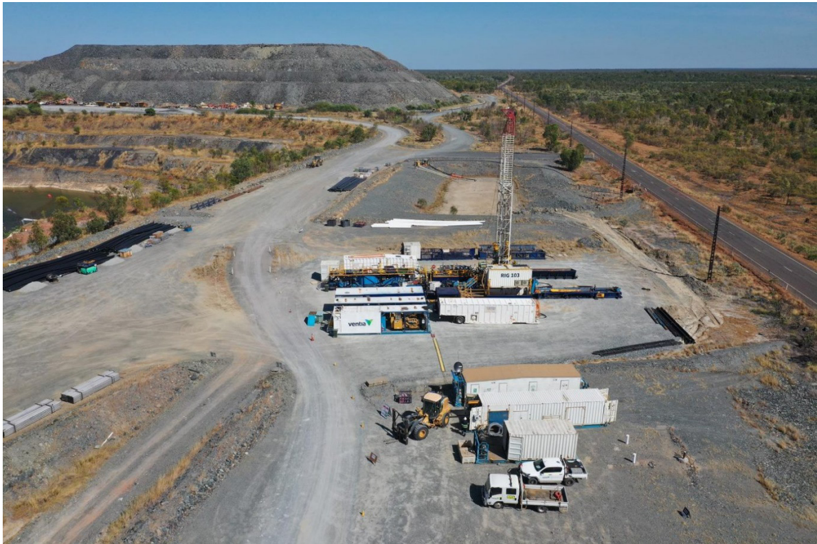
Plate ES13 Directional drilling for brine injection into Pit 3 underfill (2022)
