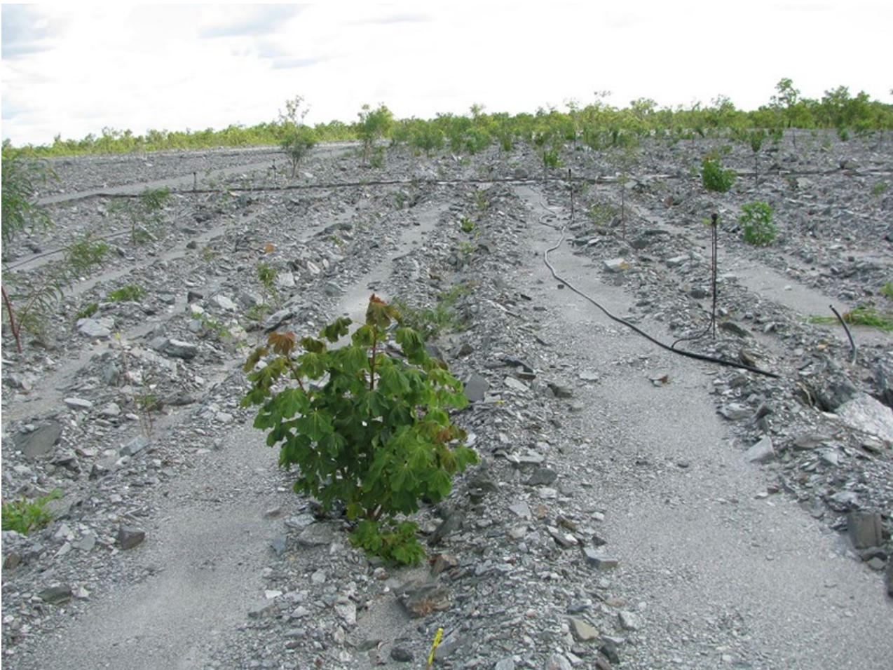
Photo 1: Contour ripping on trial landform trial of 2 m interval (2010)
