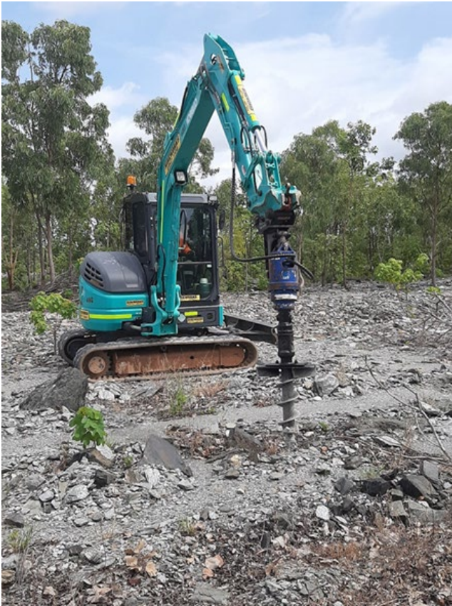
Photo 4: Small excavator with auger attachment
