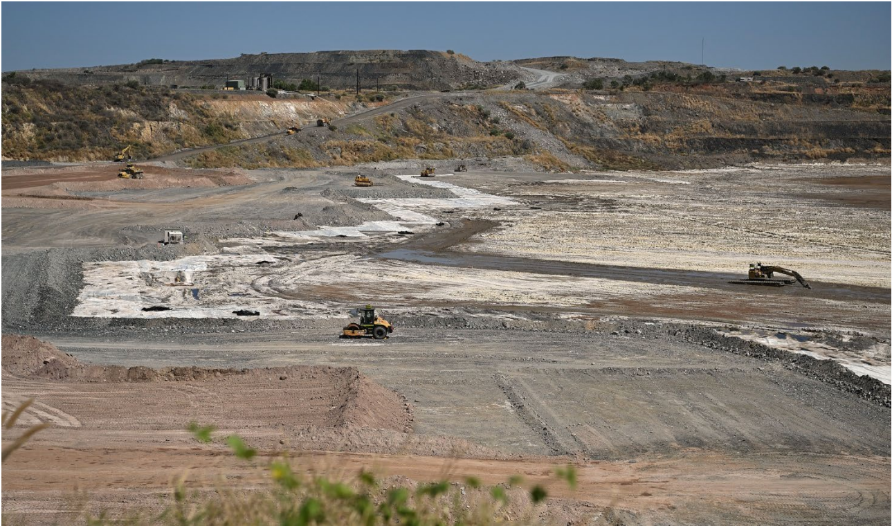
Photo 14: Installation of geotextile and construction of initial capping on Pit 3 (2025)
