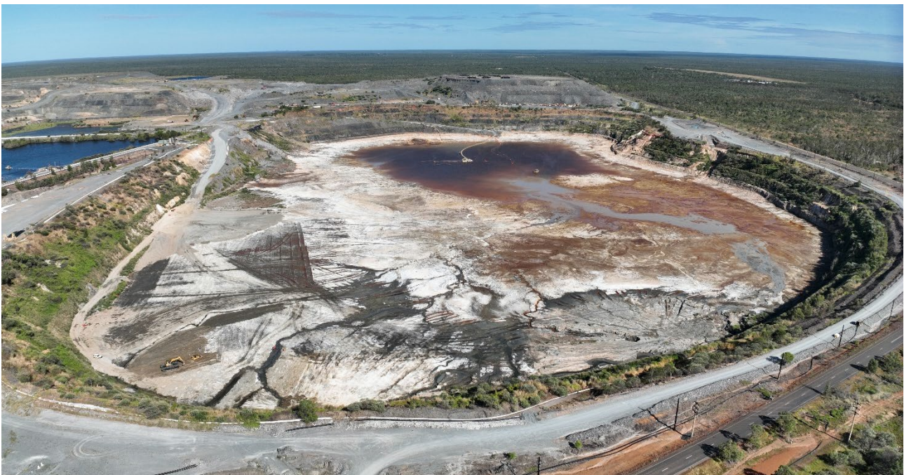
Photo 13: Dewatering Pit 3 (April, 2024)
