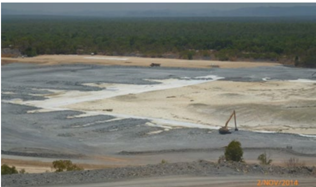
Photo 5: Pit 1 being backfilled (2014)
