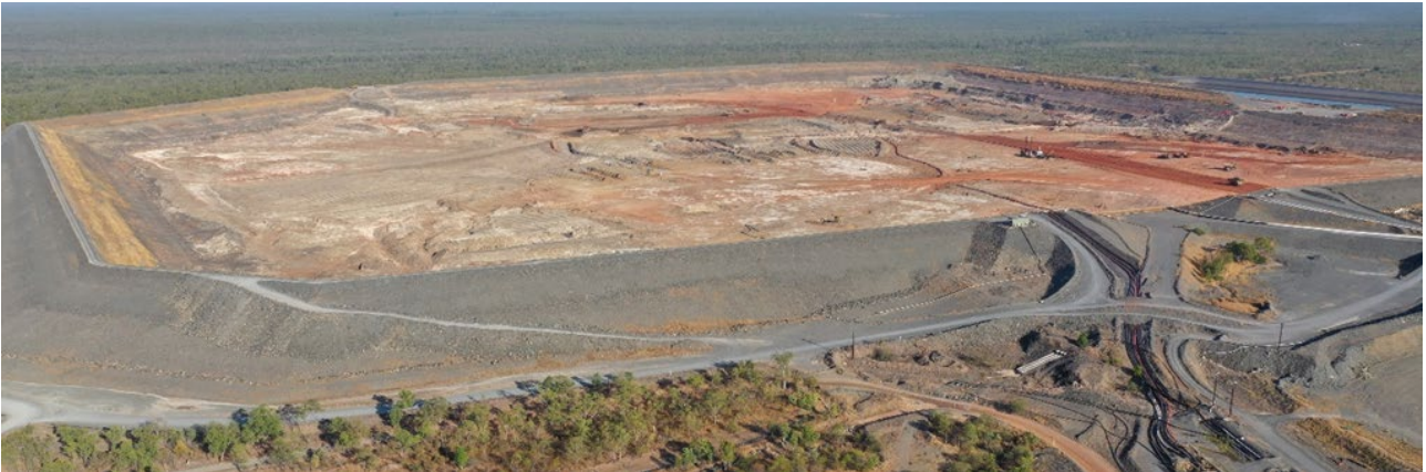
Photo 16: Ranger Water Dam in final stages of remnant tailings removal from floor (2021)
