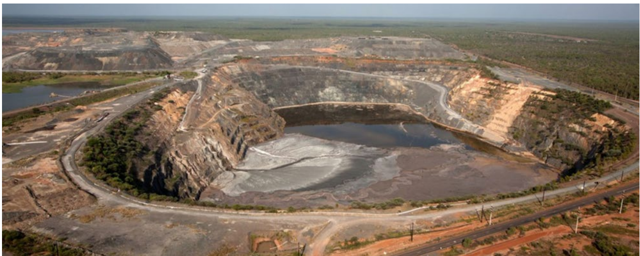
Photo 11: Pit 3 tailings deposition (2016)
