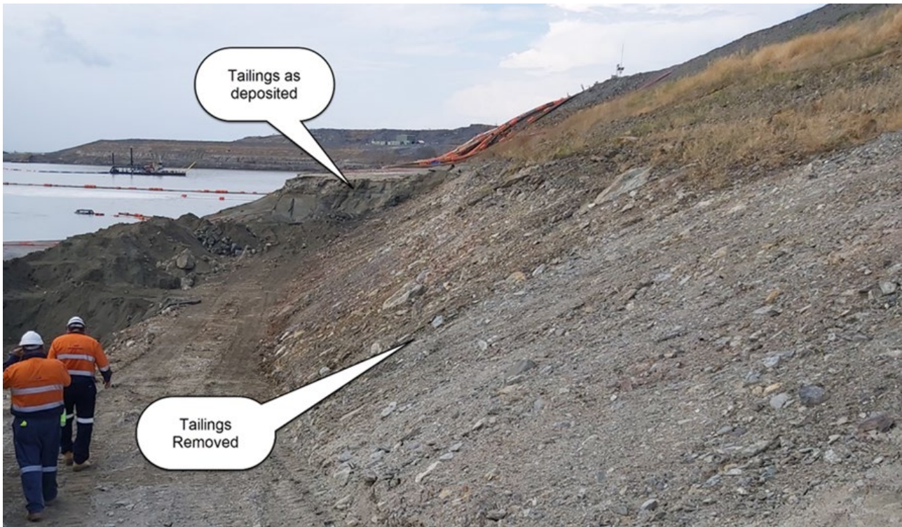
Plate 14: Cleaning remnant tailings from walls of tailings storage facility (2020)
