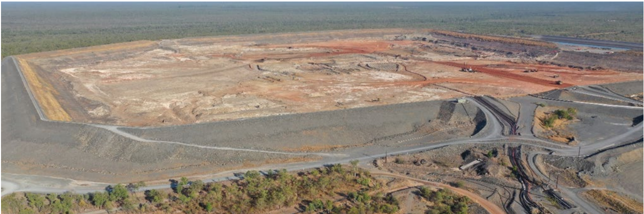
Plate 15: Ranger Water Dam in final stages of remnant tailings removal from floor (2021)
