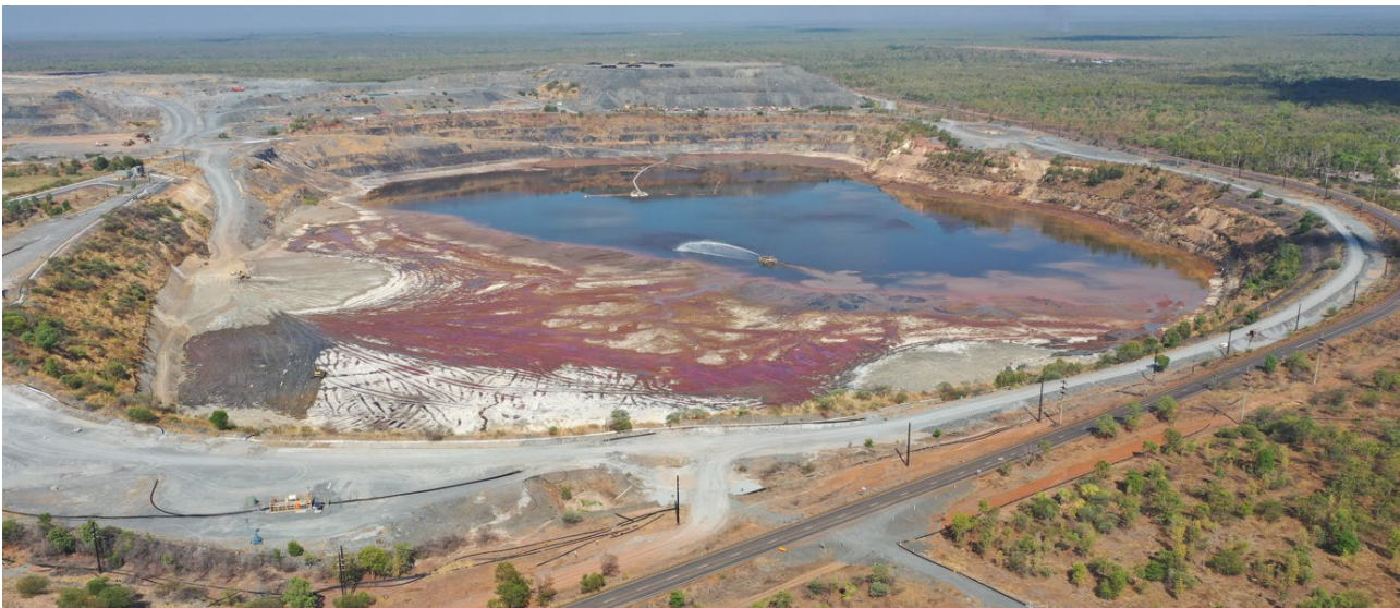
Plate 13: Dewatering Pit 3 (November, 2023)
