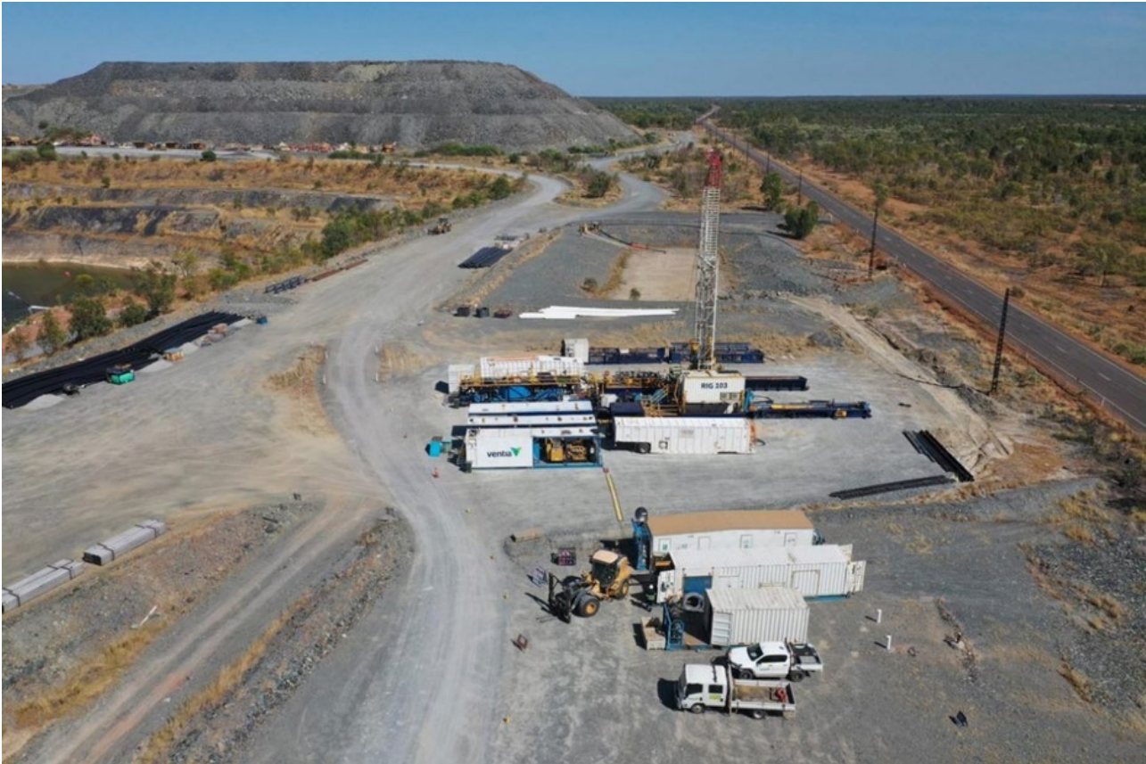
Plate 12: Directional drilling for brine injection into Pit 3 underfill (2022)
