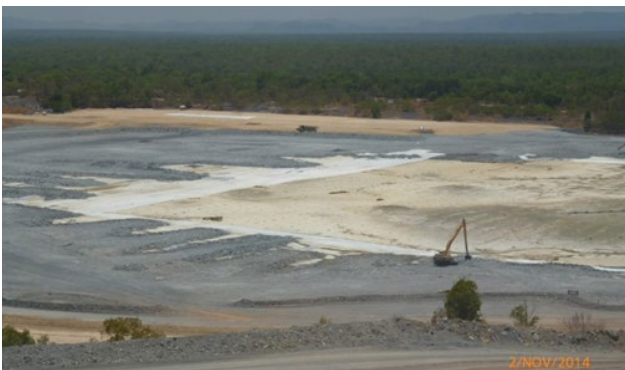
Plate 5: Pit 1 being backfilled (2014)
