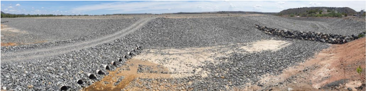
Plate 8: Pit 1 perimeter drain with access track (left) and rock check dam (right) (2021)
