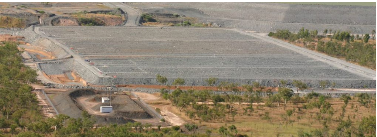
Plate 17: Trial landform constructed (2009)
