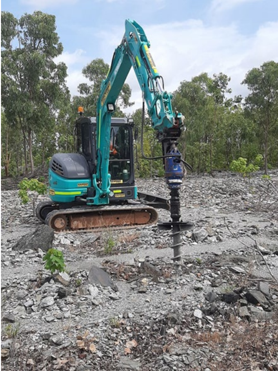
Plate 1: Small excavator with auger attachment
