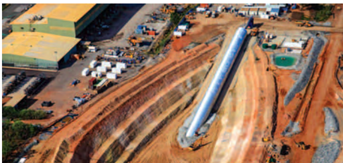
Figure 9-83: Boxcut and portal, completed in December 2012
