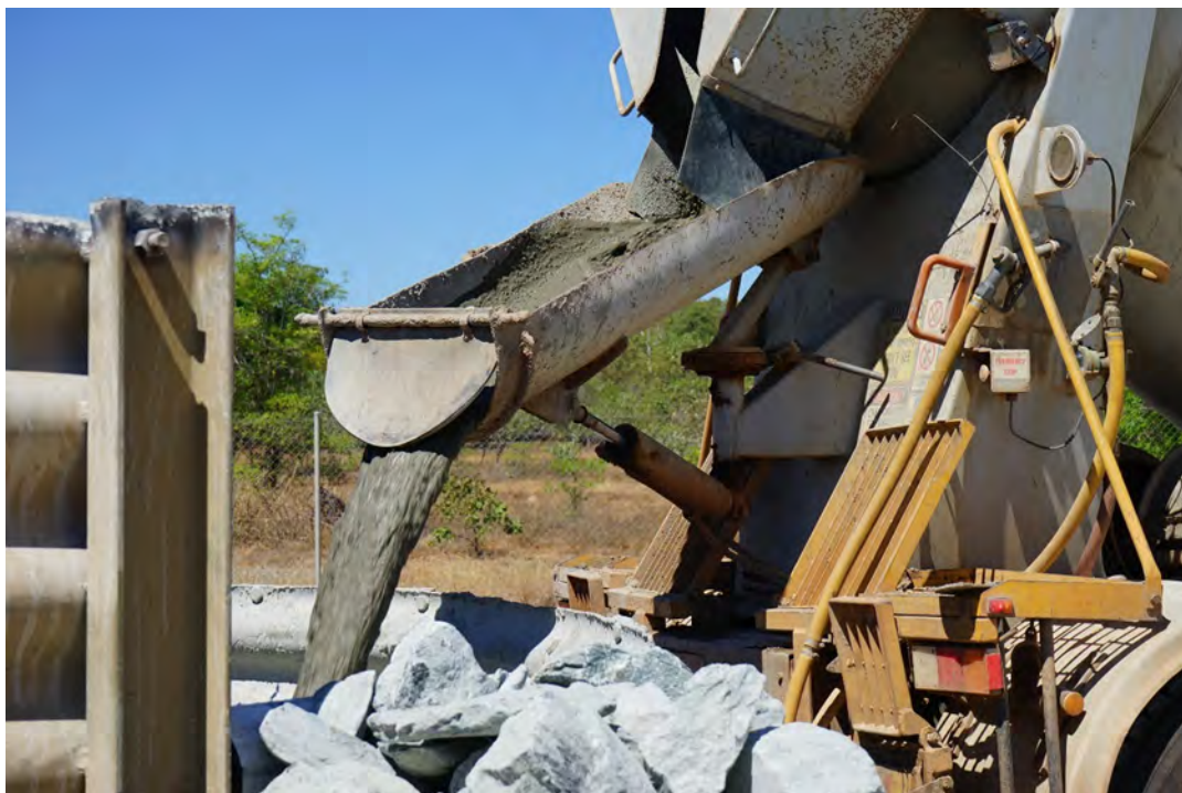
Figure 9-89: Cement slurry being added to the rockfill at ventilation shaft to create the CRF plug (ERA 2022)
