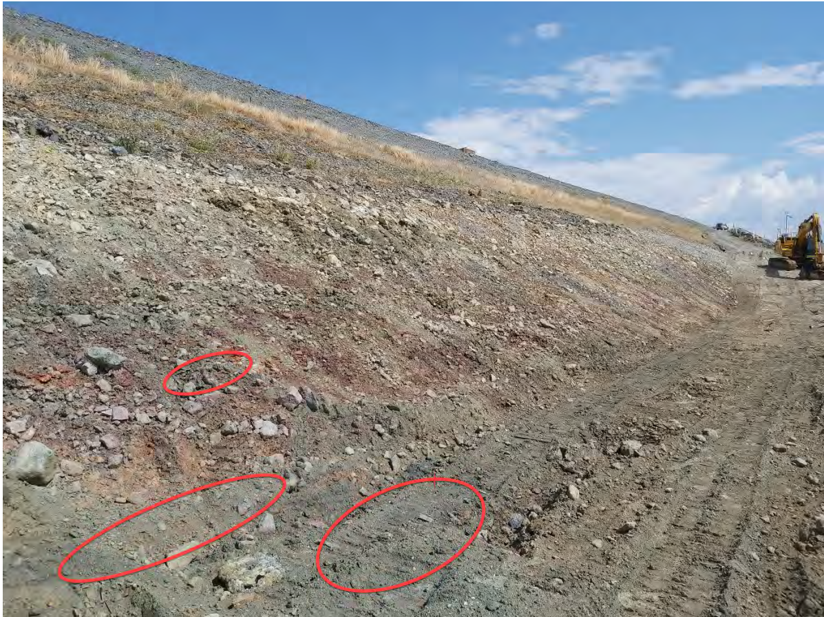
Figure 9-62 –RWD wall post step 1 & 2, with tailings patches indicated (dark grey/khaki colour)
