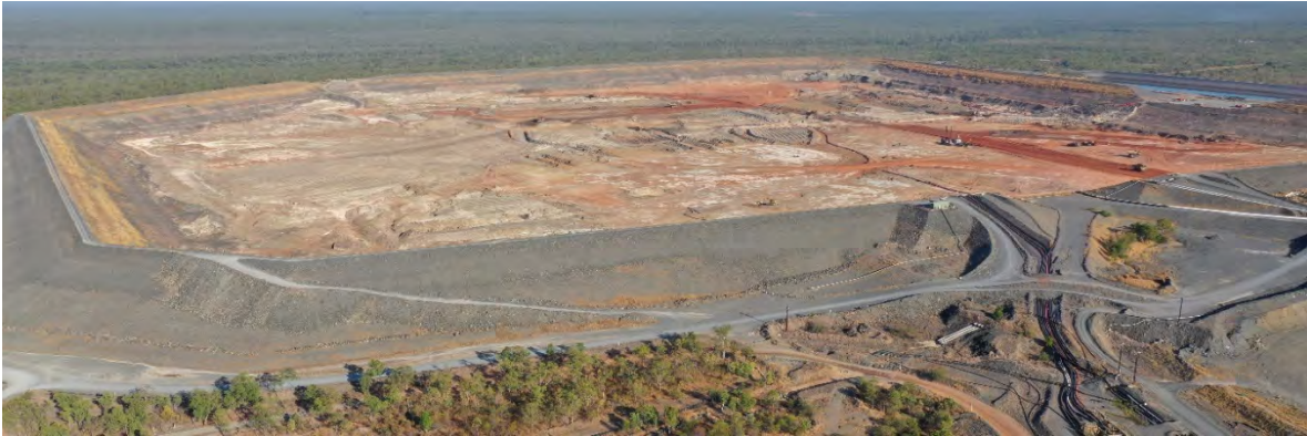
Plate ES15: Ranger Water Dam in final stages of remnant tailings removal from floor (2021)
