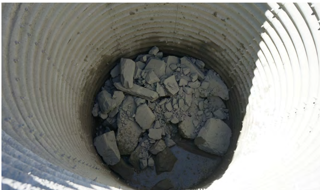
Figure 9-90: Top of CRF plug in the vent shaft to 4 m below surface (ERA 2022)
