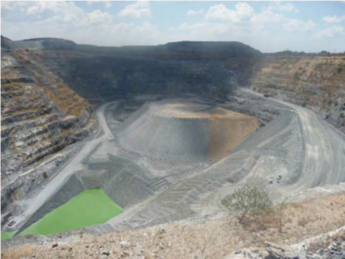
Figure 9-16 Pit 3 underfill during construction in 2014
