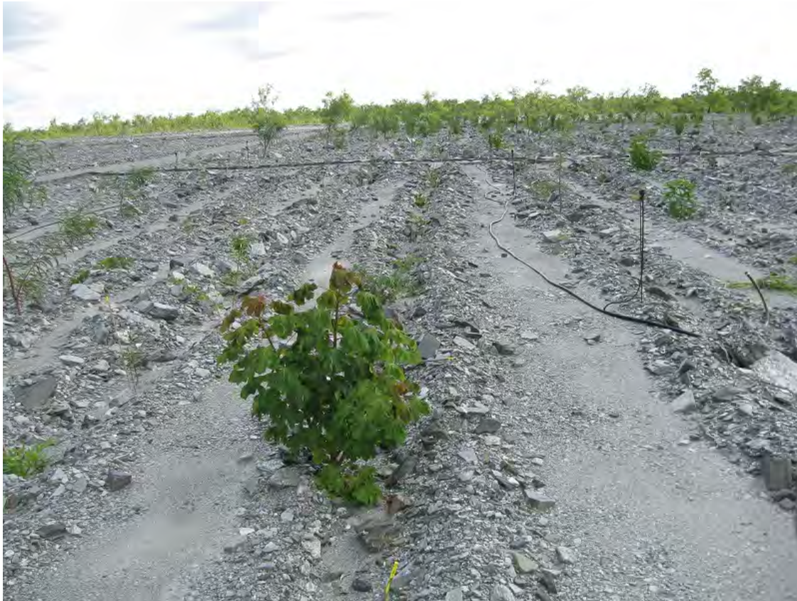
Figure 9-118: Contour ripping on trial landform trial of 2m interval (2010)
