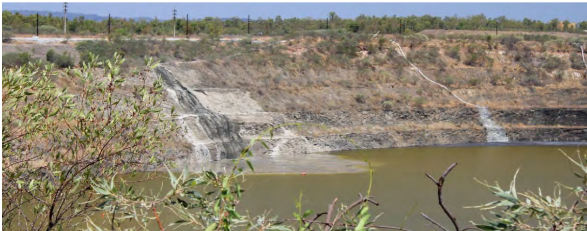
Figure 9-20 Southeast wall of Pit 3 - subaerial discharge point for mill tailings (November 2019)
