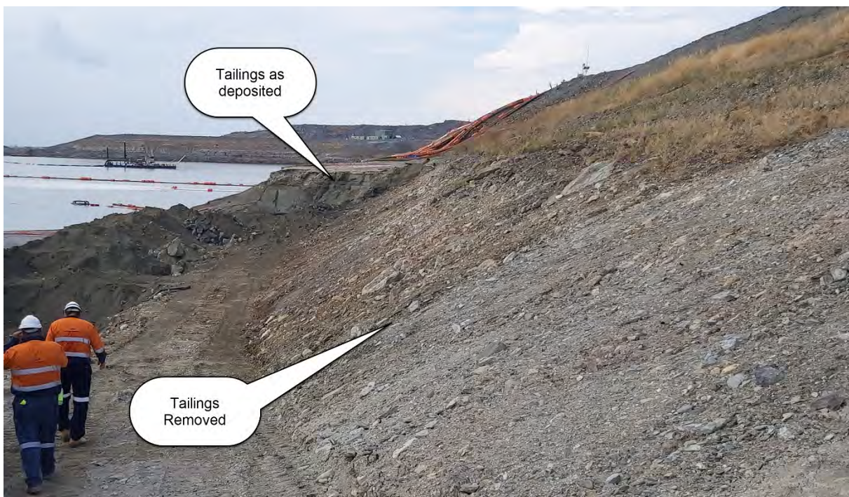
Figure 9-61 Typical wall cleaning operation above 45 mRL
