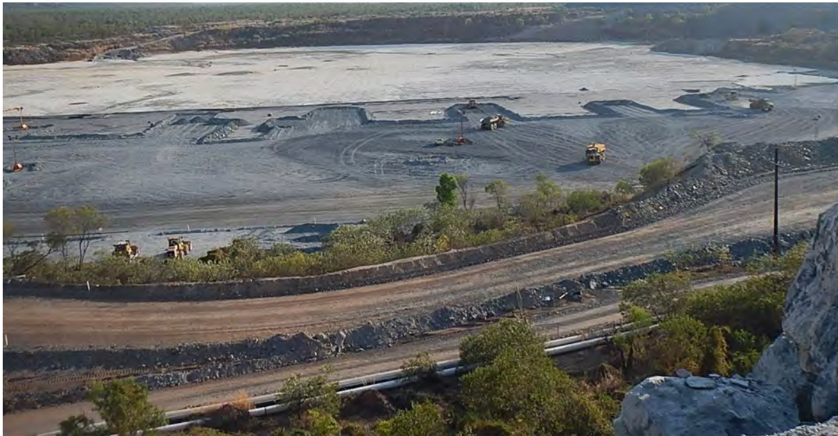
Figure 9-43 Pit 1 Capping construction method showing material 'fingers' pushed across the geotextile.
