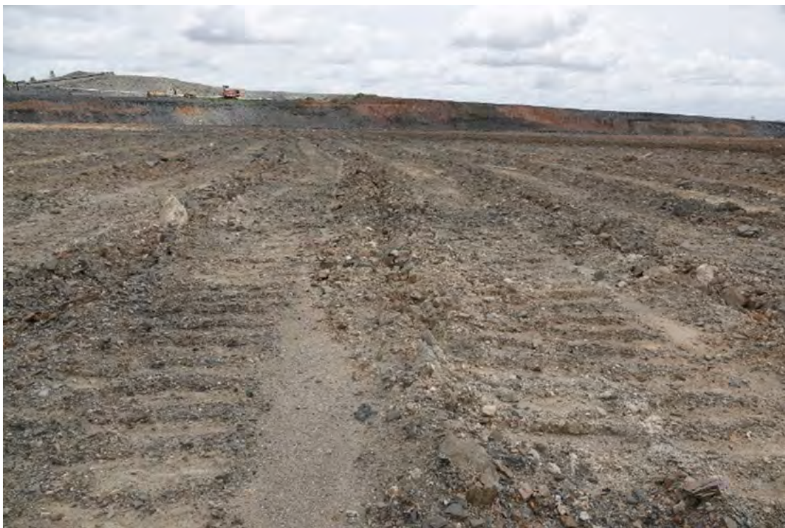
Figure 9-119: Contour ripping on Stage 13, with 3 m intervals (March 2020)
