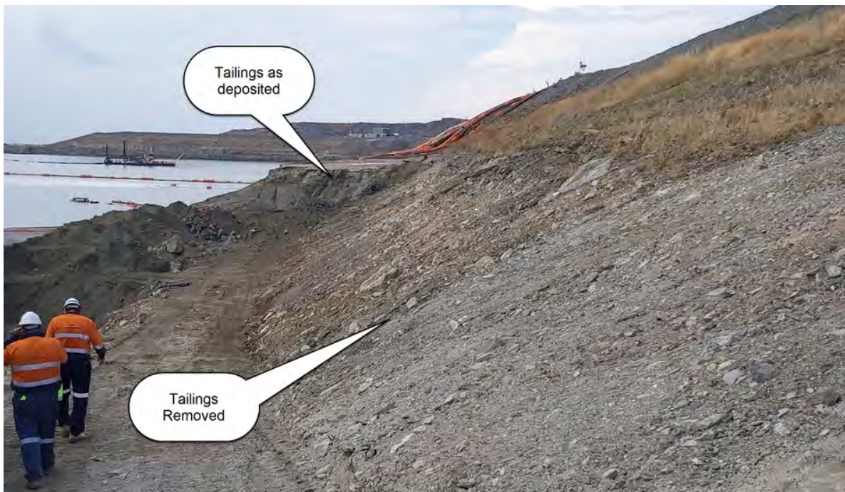
Plate ES14 Cleaning remnant tailings from walls of tailings storage facility (2020)
