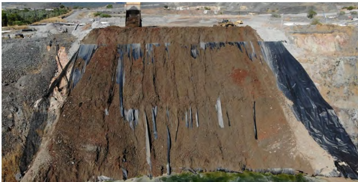
Figure 9-31 Transfer of tailings down tip head in Pit 3
