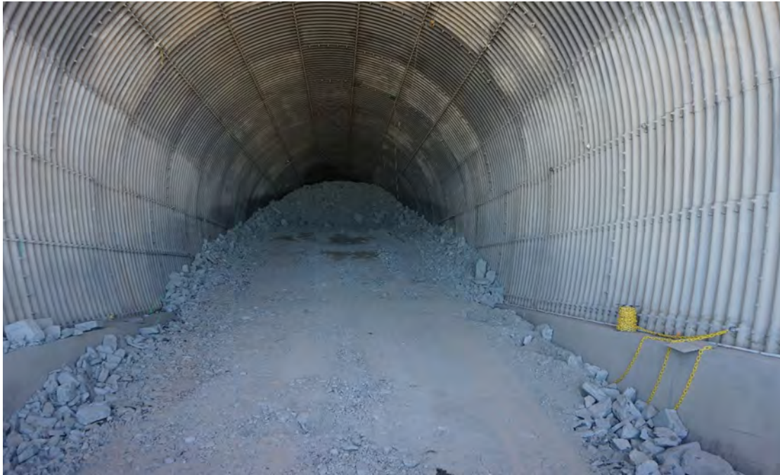
Figure 9-87: Picture taken after completion of backfilling to 22 mRL, (CL 06 m) with a total of 29,015 t waste rock placed (ERA 2022)
