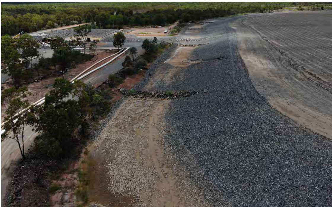
Figure 9-7: View of the perimeter drain along the southeast edge of Pit 1 (January 2021)
