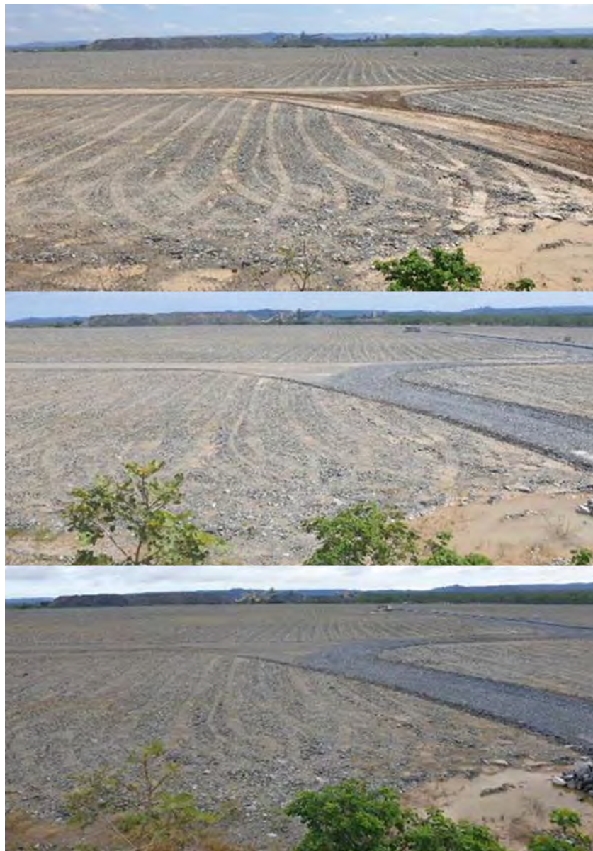
Figure 9-5 Scarification as seen on 28 Oct 2020 (top), 6 Jan 2021 (middle), 17 Feb 2021 (bottom)
