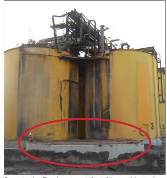
Deconstruction: The cleared area in front of the remaining leach tanks, with the base of Leach Tank 1 circled in red following its removal
