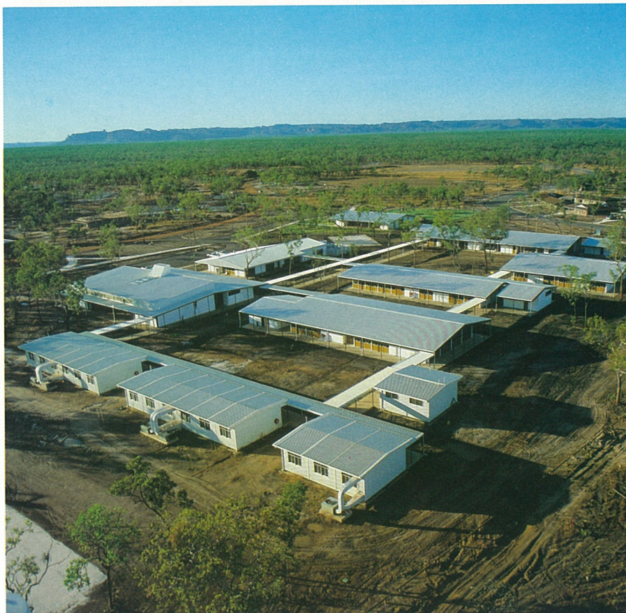
Left School buildings at Jabiru are already being used. Right The new Jabiru town is bordered by a man-made lake.
