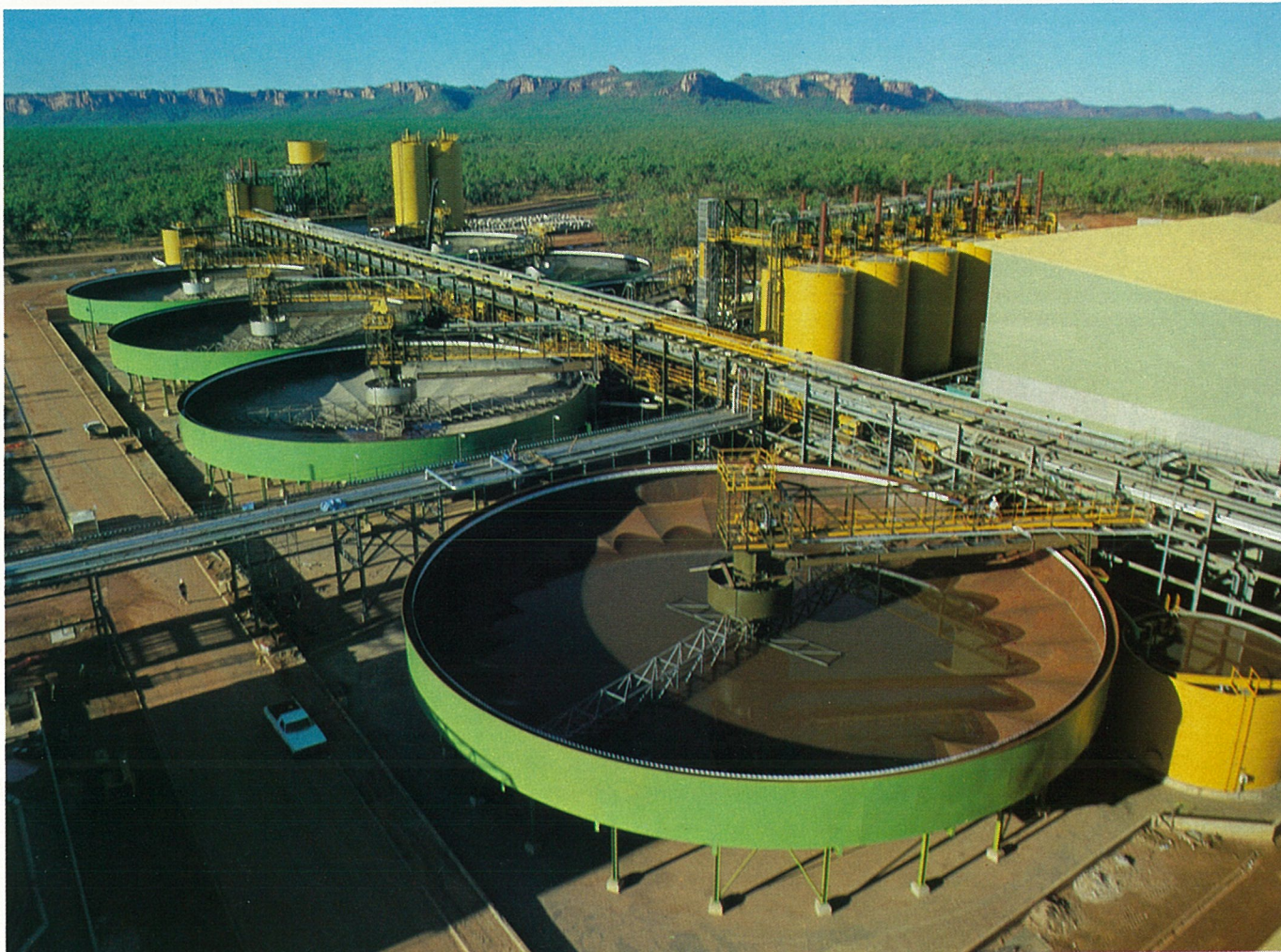
Above The plant with counter-current decantation thickeners in foreground, and Mount Brockman in far distance.
