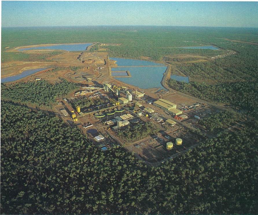
Water management forms an extensive part of the Ranger operation, involving a tailings dam and system of retention ponds.
