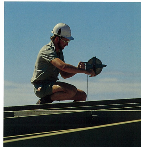
Below (lower): Senior Mill Engineer Warren Lofthouse inspecting floor of thickener.
