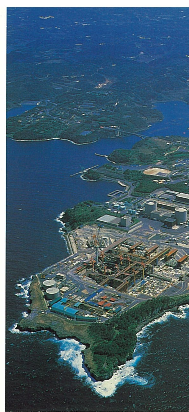
The Genkai nuclear power plant in Japan operated by Kyushu Electric Power Co.
