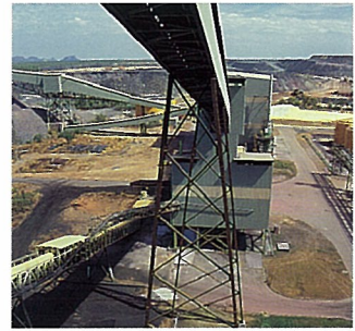
Above: Conveyors leading from the Ranger crushing plant.
