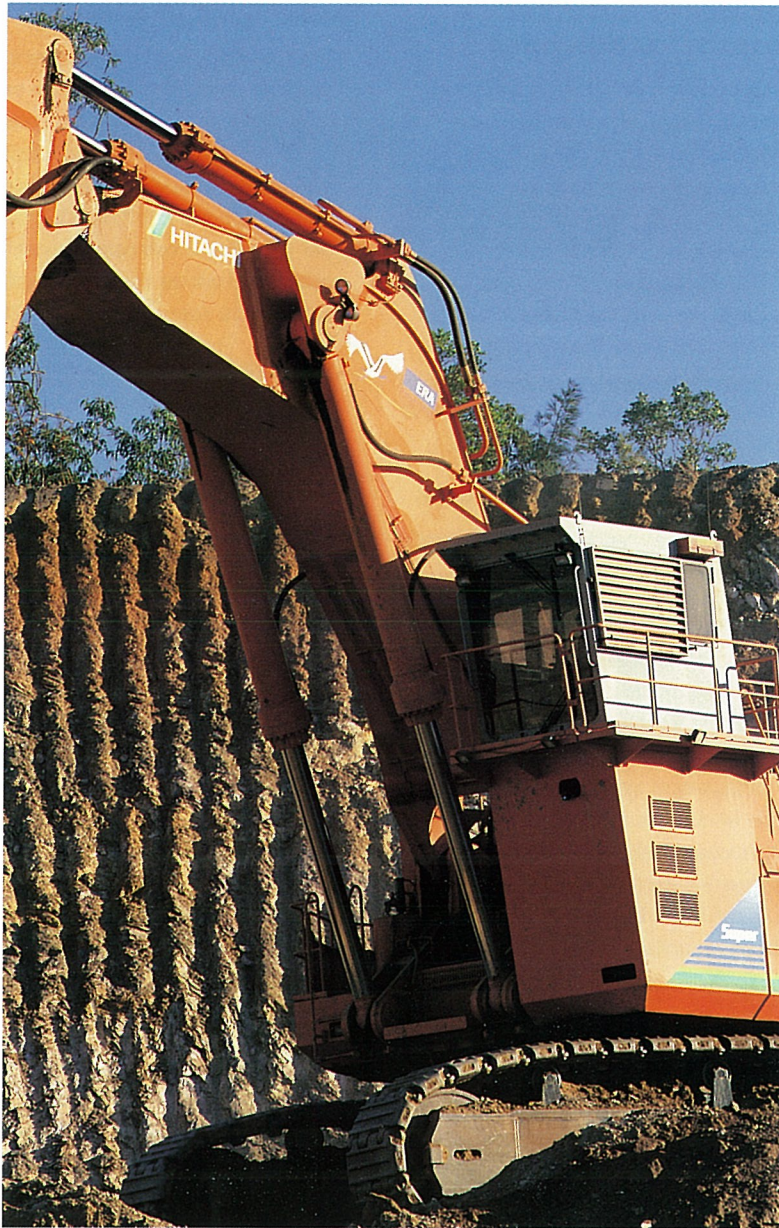
Excavation work in the pit area of Ranger #3.
