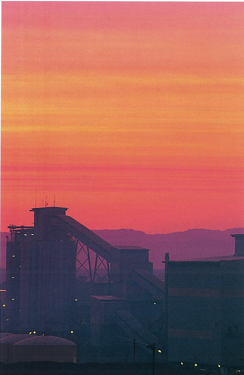
Morning light engulfs the processing plant at Ranger. The plant capacity expansion was fully commissioned during the year.
