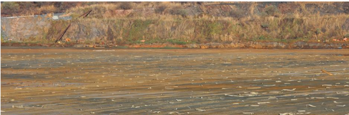
Plate 4-3: Tailings surface showing tops of vertical wick drains installed in Pit 1
