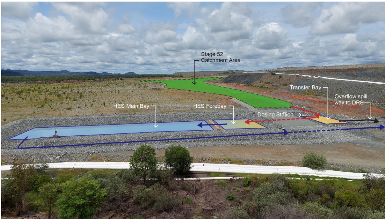
Plate 6-2: Stage 52 HES Basin (31 January 2023)
