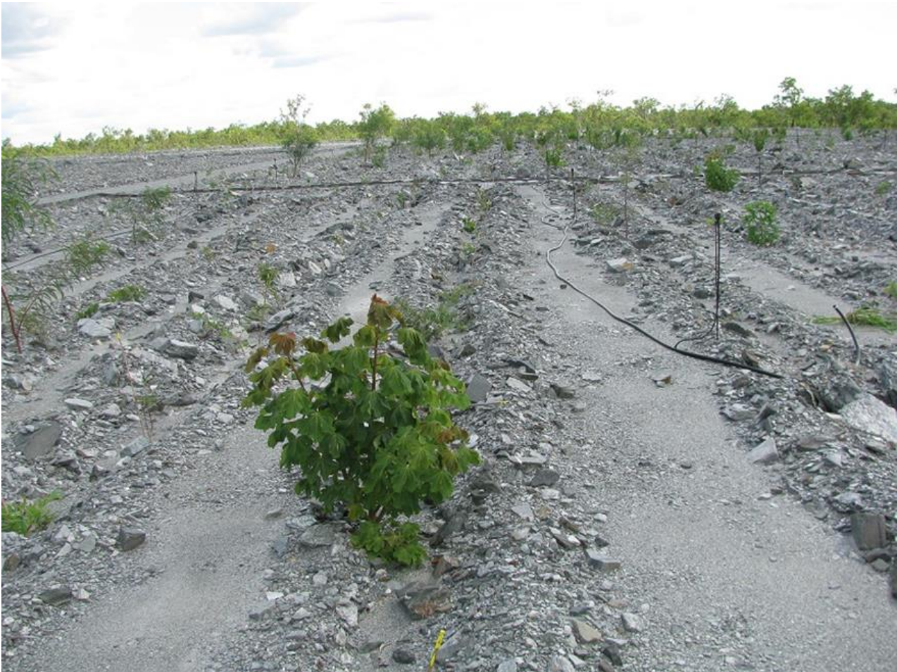
Plate 9-1: Contour ripping on trial landform trial of 2 m interval (2010)
