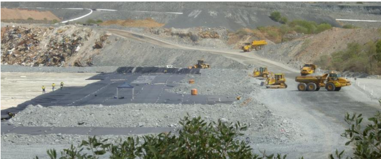
Plate 4-14: Installation of geotextile, construction of groynes and initial capping on Pit 1
