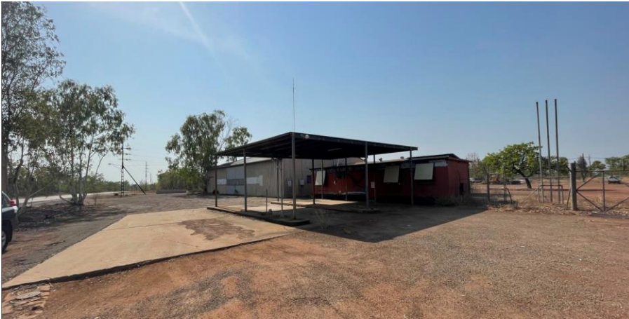
Plate 4-23: Gagudju workshop and surrounding infrastructure
