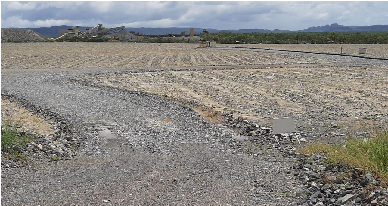
Plate 4-4: Scarification of the surface on Pit 1 (October 2020)
