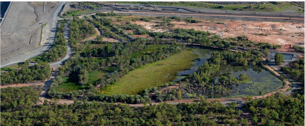
Plate 4-17: Corridor Creek Wetland Filter (CCWLF)
