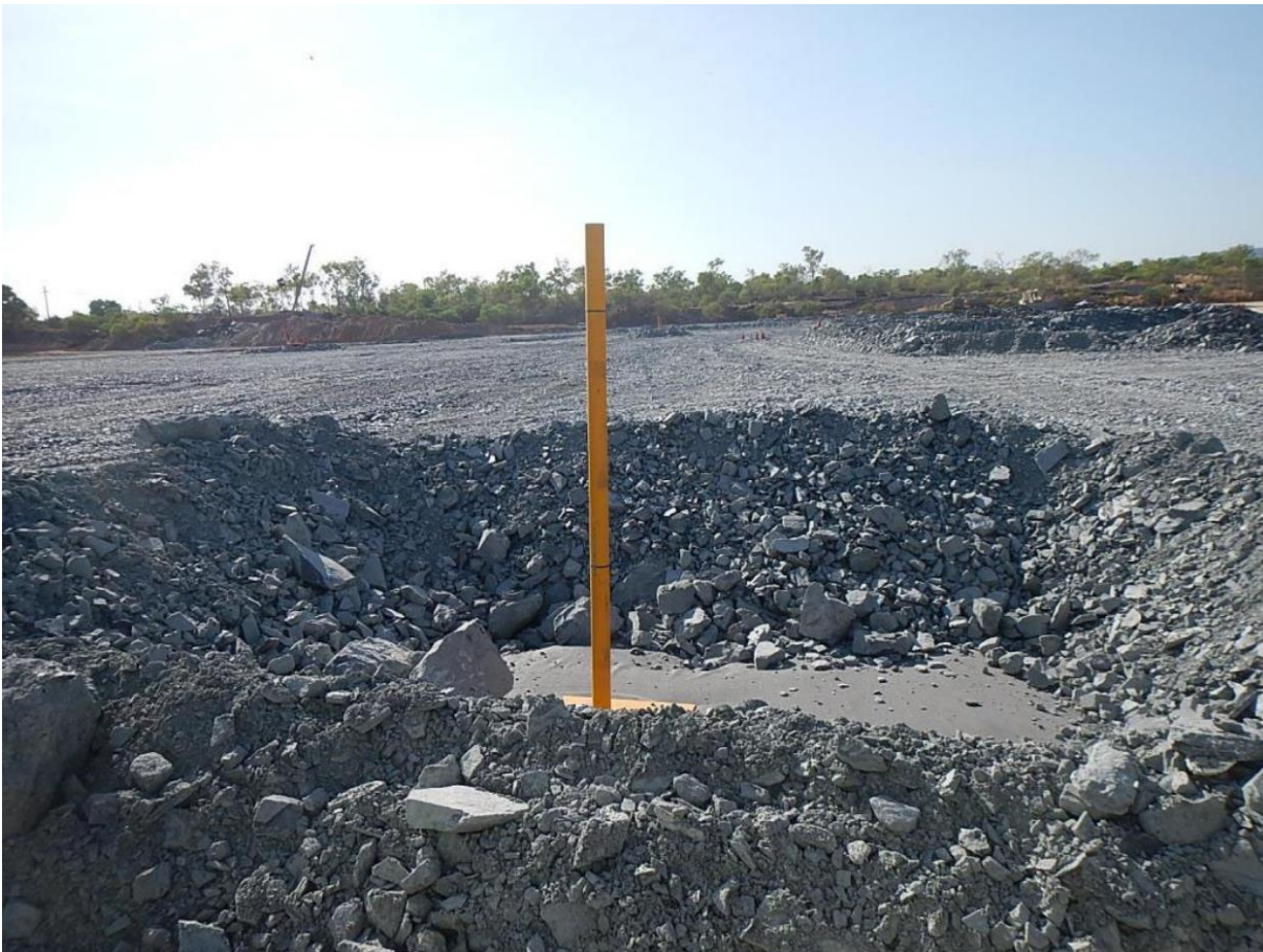
Plate 4-2: Settlement monitoring plate, with standpipe, at time of installation
