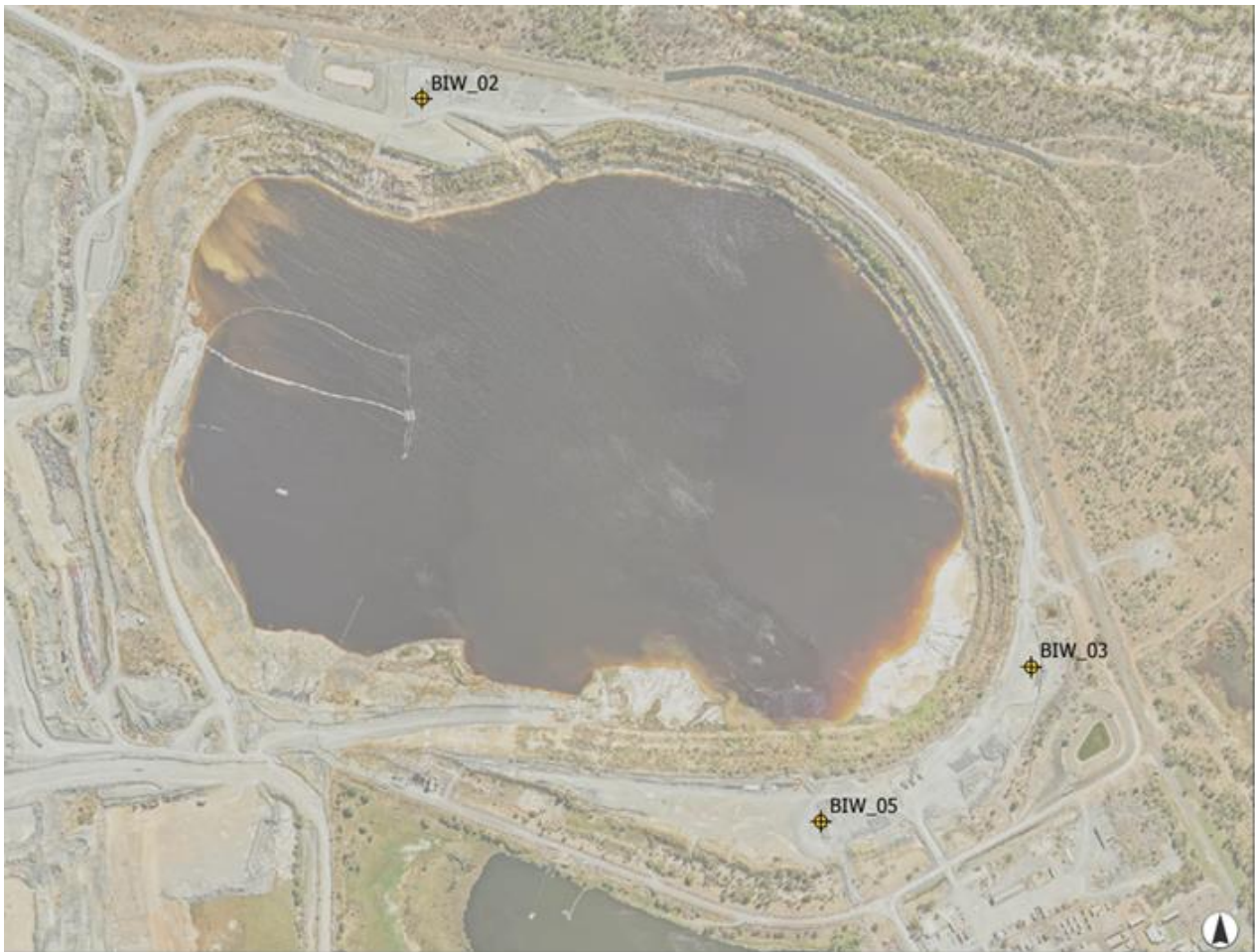
Figure 4-9: Location of Well Heads of the Directionally Drilled Brine Injection Wells
