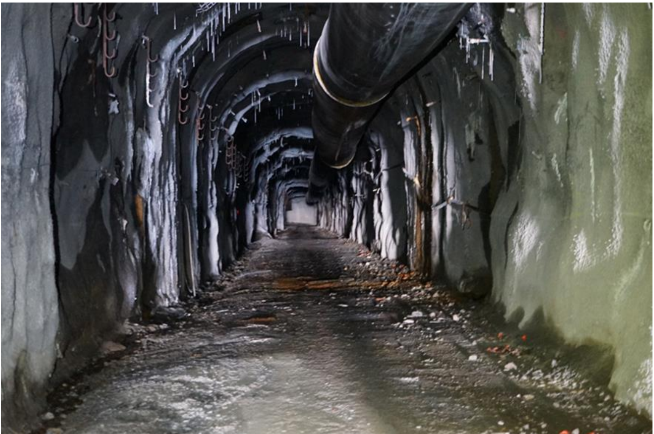
Plate 4-30: The end of the steel multiplate tunnel (June 2022)
