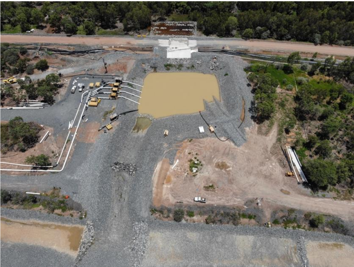
Plate 4-6: Completed Corridor Road Sump upgrade works with pumping infrastructure installed
