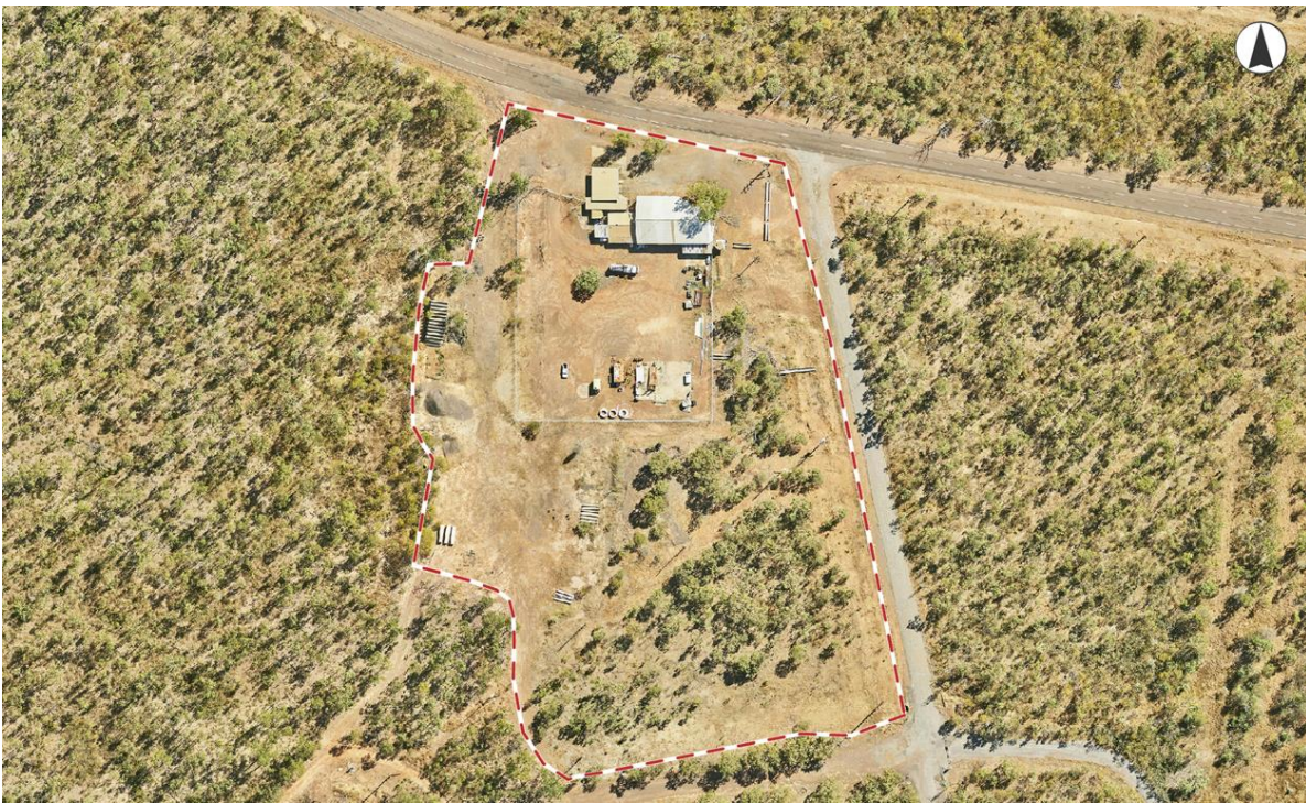
Plate 4-22: Gagudju yard and surrounding disturbance (June 2023)
