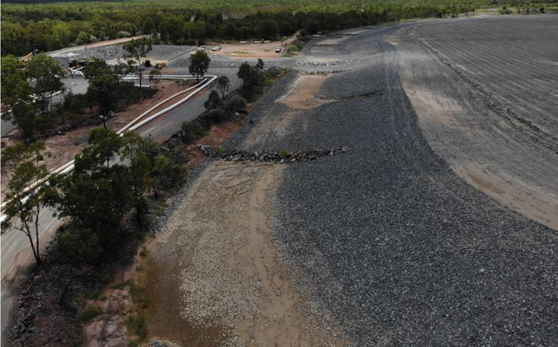
Plate 4-5: View of the perimeter drain and rock check dams along the southeast edge of Pit 1 (January 2021)
