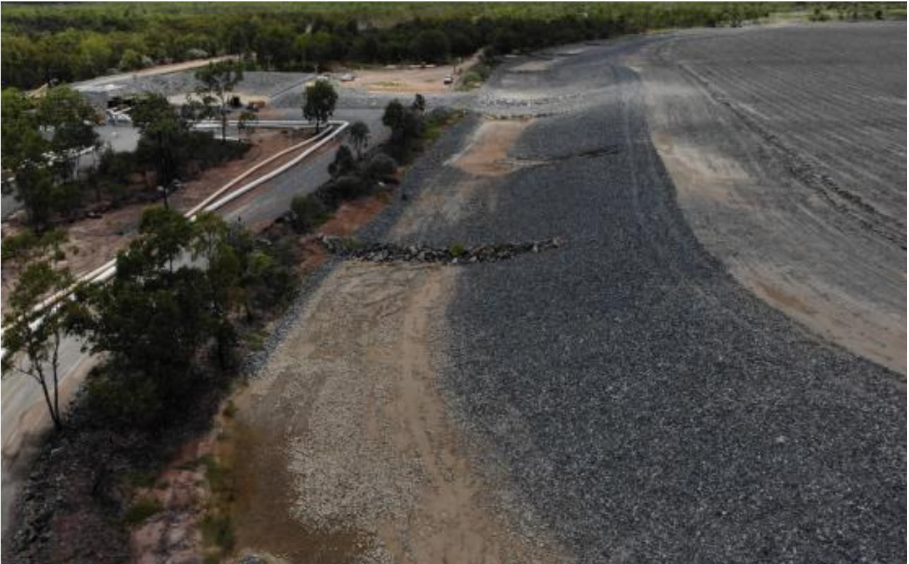
Plate 6-1: Pit 1 perimeter drain
